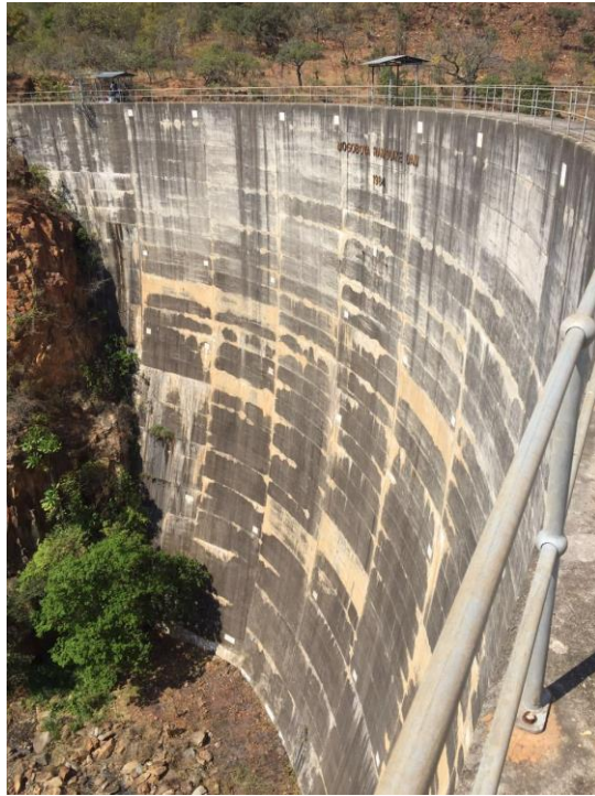
Figure 6-6: General view of the downstream face of the arch
