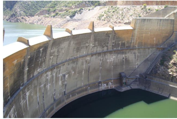
Figure 2-21: Kouga Dam as viewed from the right flank (Hattingh, 2011)
