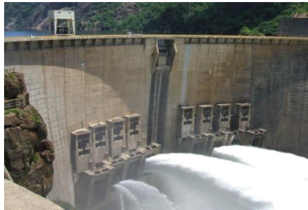
Figure 2-19: Close-up view of Cahora Bassa Dam from the downstream side (Botha et al. , 2016: 2a-210)
