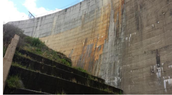
Figure 5-16: Poortjieskloof Dam: General view of the right flank downstream face
