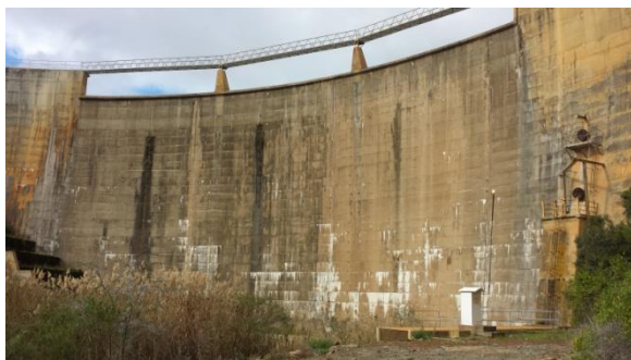
Figure 5-12: Poortjieskloof Dam: General view of spillway downstream face
