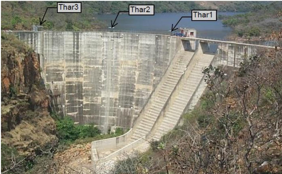
Figure 6-17: The positions of the Trivec boreholes at Thabina Dam
