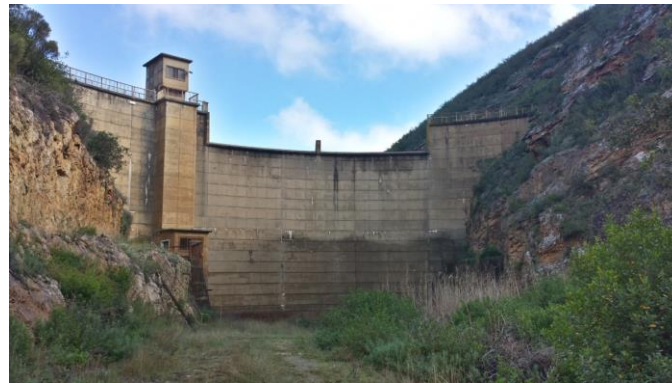
Figure 4-1: Hartebeeskuil Dam as viewed from the downstream side
