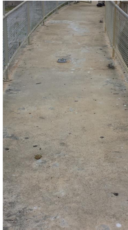
Figure 5-5: Poortjieskloof Dam: The left flank NOC
