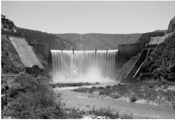
Figure 2-20: Kouga Dam as viewed from the downstream side (Mahlabela & Oosthuizen, 2012: 233)
