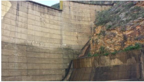
Figure 4-15: Hartebeeskuil Dam: Spillway and left flank downstream face
