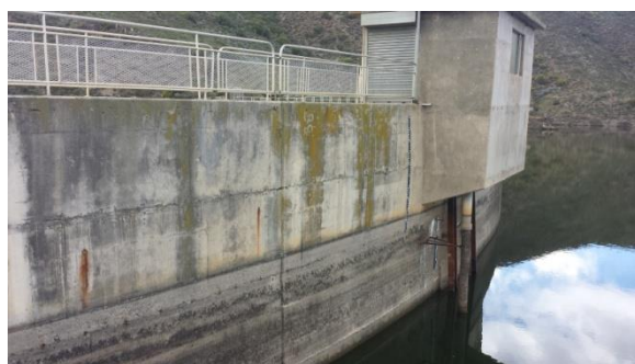
Figure 5-2: Poortjieskloof Dam: General view of left flank upstream face
