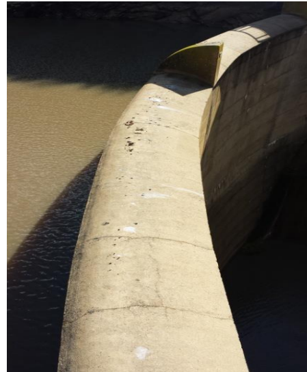
Figure 4-13: Hartebeeskuil Dam: General view of the spillway crest
