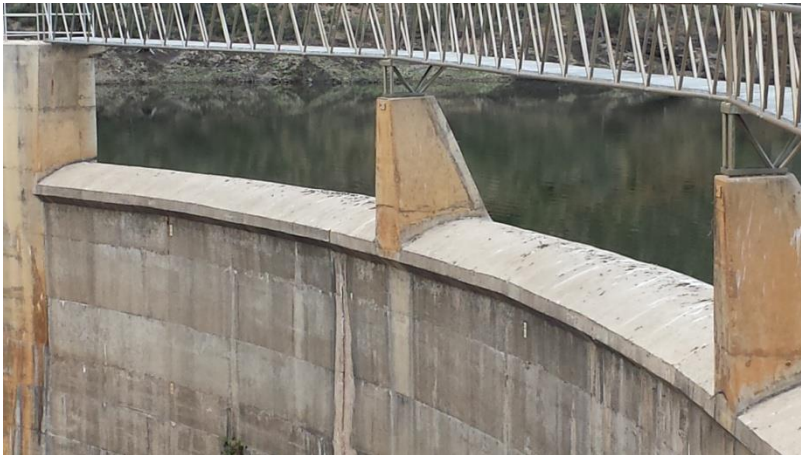
Figure 5-11: Poortjieskloof Dam: View of spillway crest
