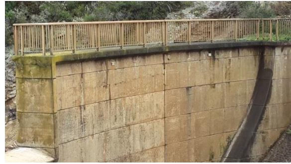
Figure 4-16: Hartebeeskuil Dam: Close-up view of left flank downstream face
