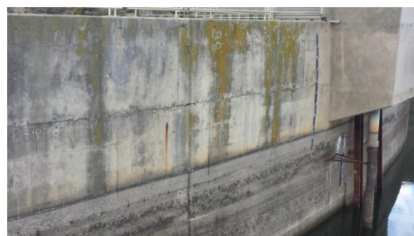
Figure 5-3: Poortjieskloof Dam: Close-up view of left flank upstream face
