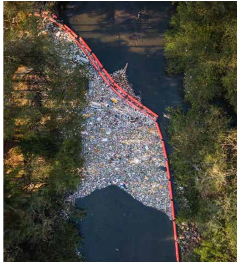
Floating garbage barriers
