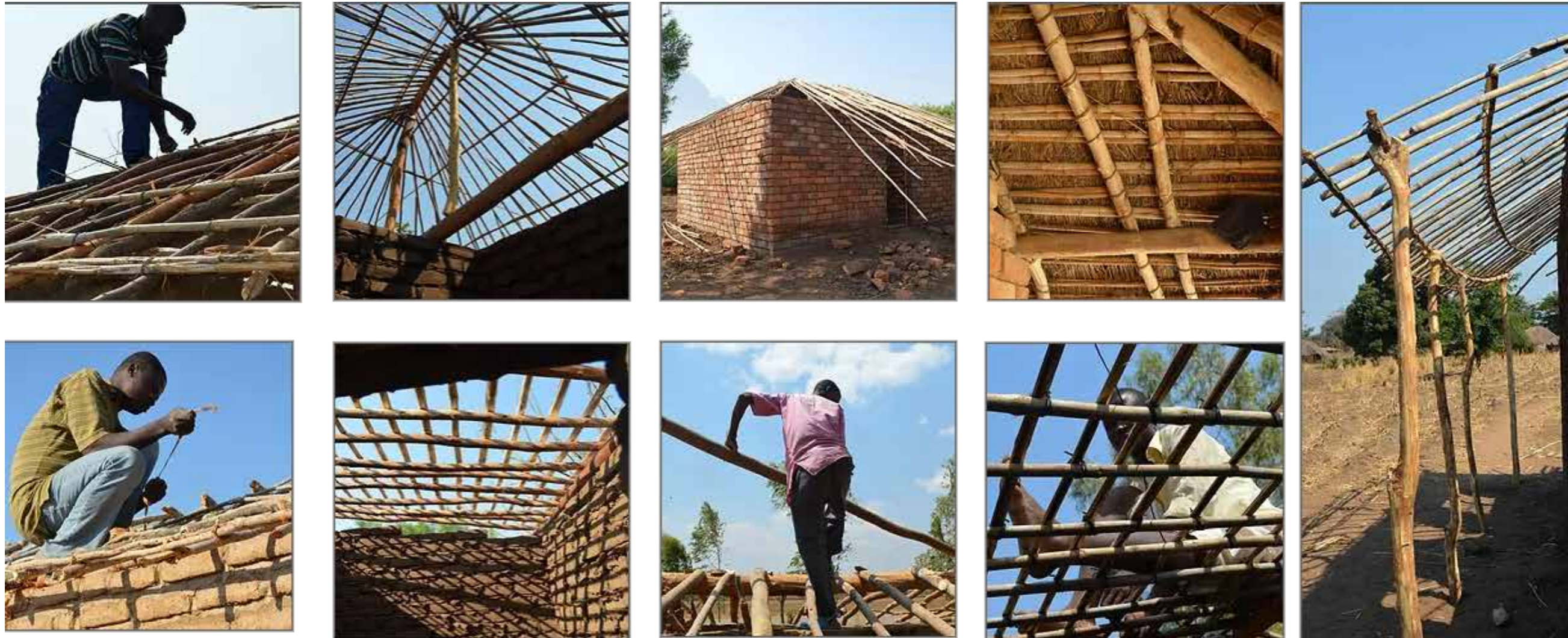
Figure 50: Construction techniques in Malawi using wooden poles and bricks (source: https://www.malawiarchitecture.com/reeds ).
