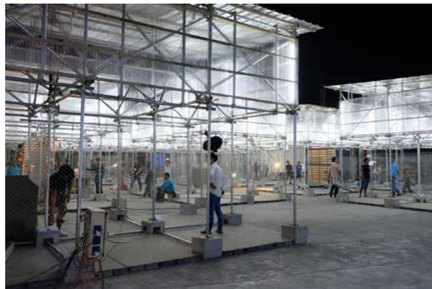
Figure 71: The steel structure forms part of the identity of the market (Gonzalez, 2018).
