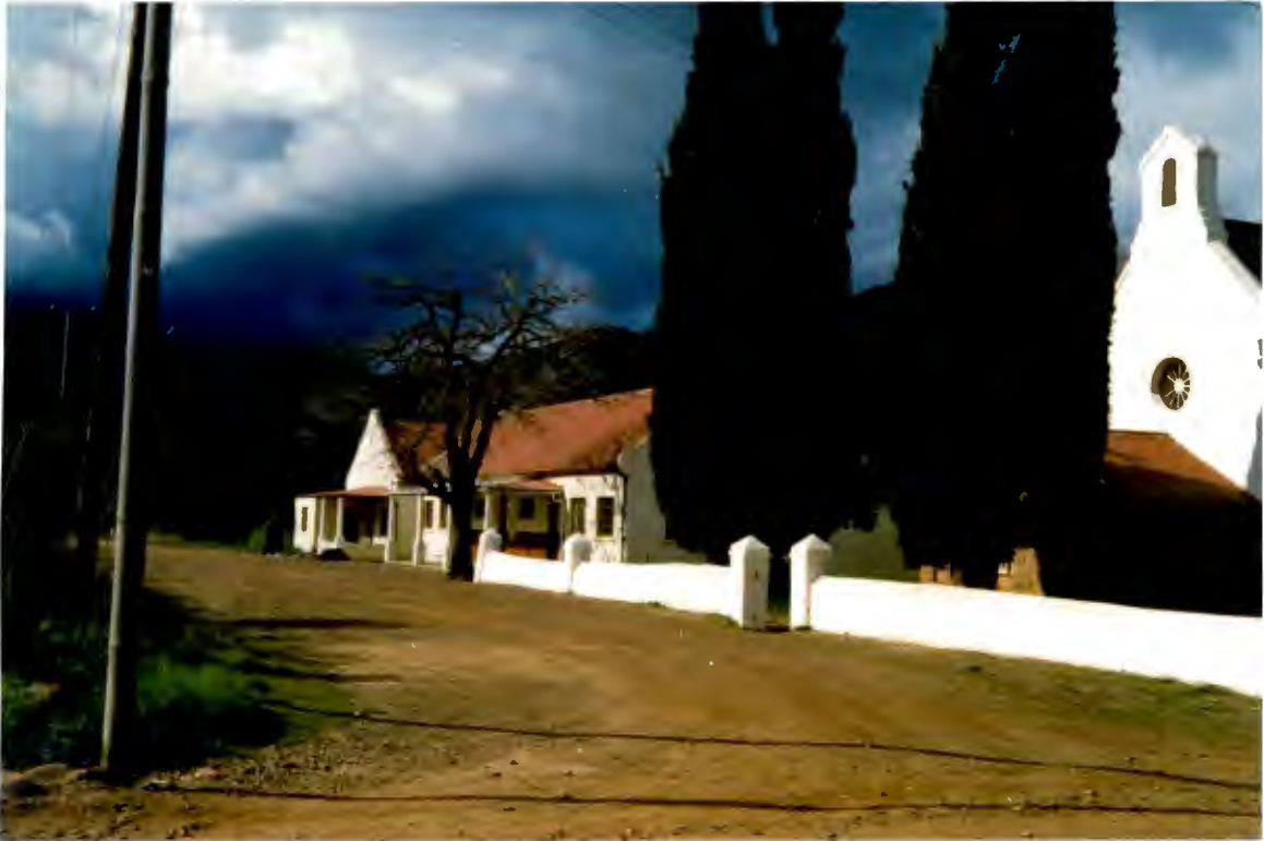
The Anglican Church School lost its thatched roof when it was rebuilt.
