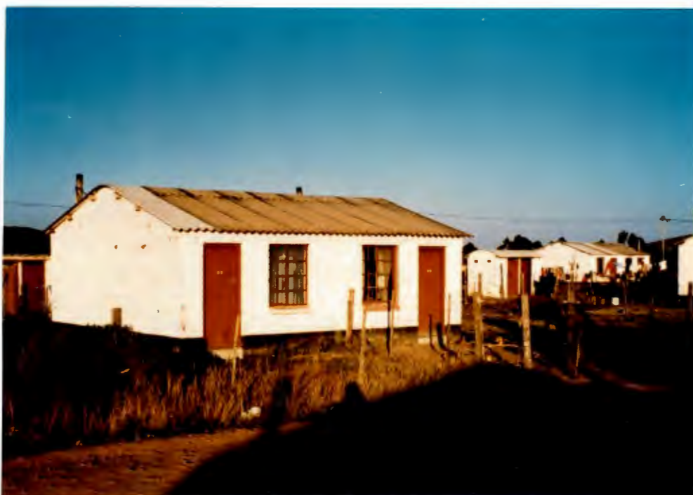
Foreground: house for two families.
