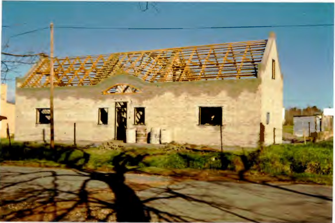
The shell of a new house under construction in Greyton in 1984.
