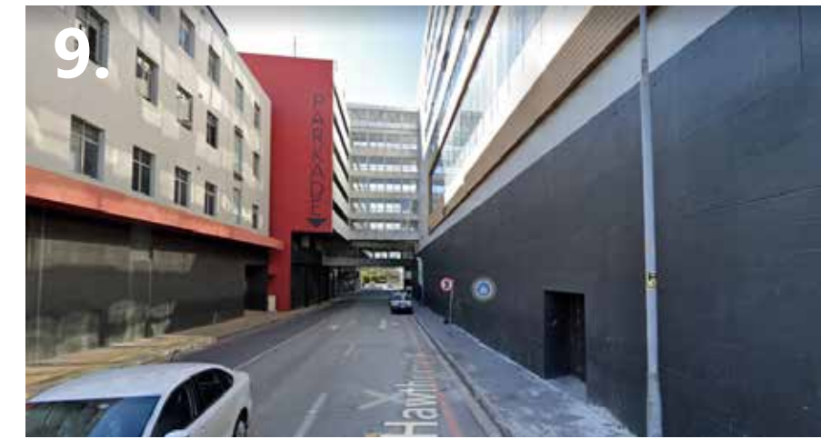
9. Hawthorne Road underpass
