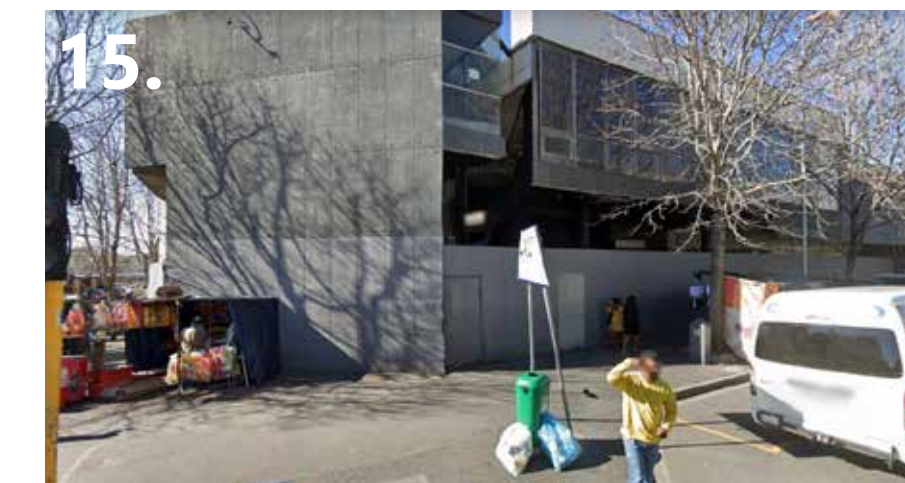
15. Newry Street & Main Road - Werdmuller current condition
