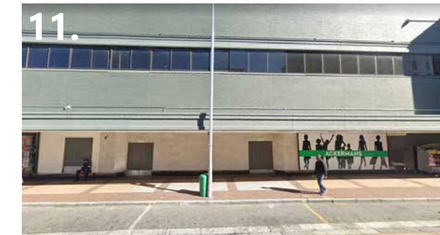
11. Main Road-towards Cavendish Square
