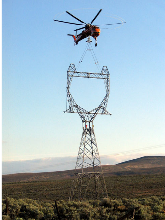
Figure 1.1.1: Erickson Aircrane placing a powerline tower (Incorporated 2013)
