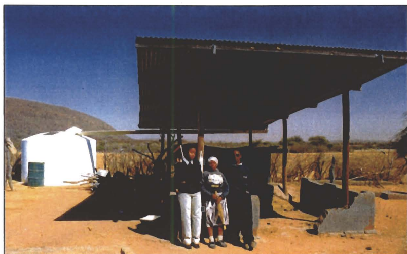
Plate 5.5: Mrs Ntebogang (centre) with members of the BTC beside the rainwater catchment roof and ferrocement tank, Kgotla lands area
