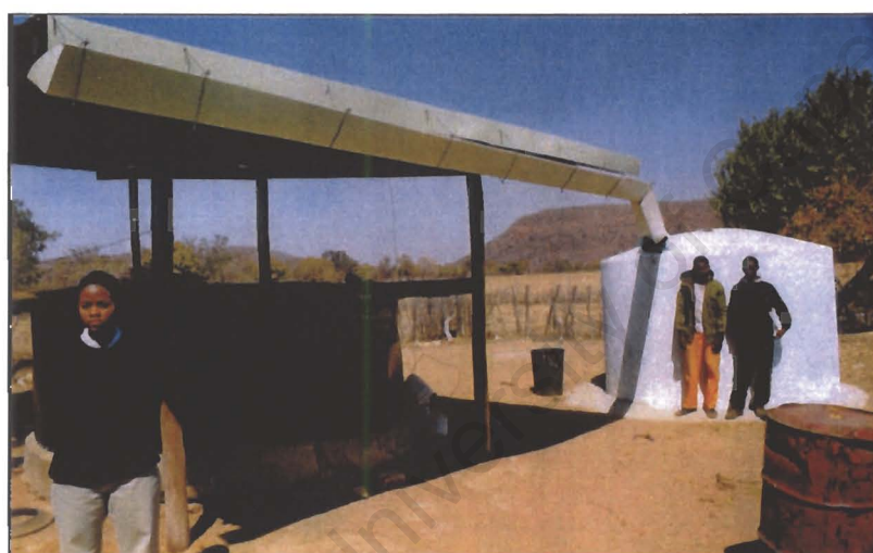
Plate 5.6: Members of the BTC beside Mr Kgopiso's (centre) rainwater catchment roof and ferrocement tank, Polokwe lands area
