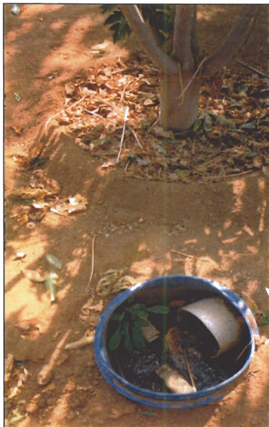
Plate 7.2: A perforated plastic drum with inlet pipes that carry waste grey household water, beside a paw paw tree in Gabane.
