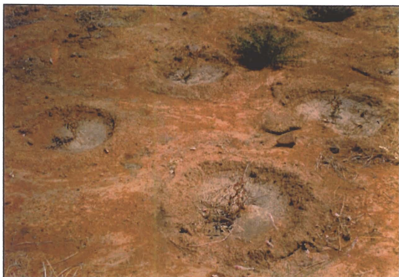
Plate 5.14: Spherical microcatchments each 0.85m in diameter with openings facing upslope to catch runoff for the Combretum species (Dry season, winter photograph)
