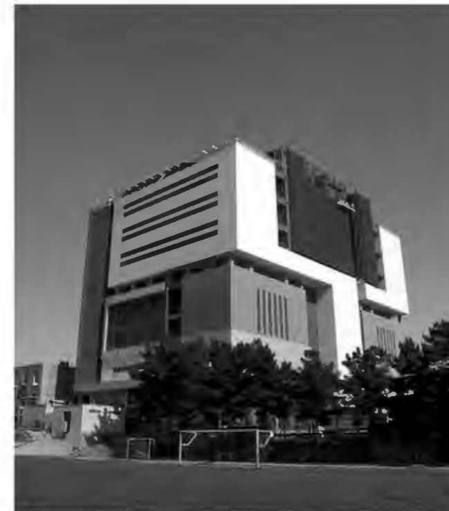
figure 83. The Telecommunication centre, located in Tehran, is an example of the influence of western architecture. From concept to selection of materiality, this building fails to embody any of the Iranian traditional ideologies or the cultural needs.
