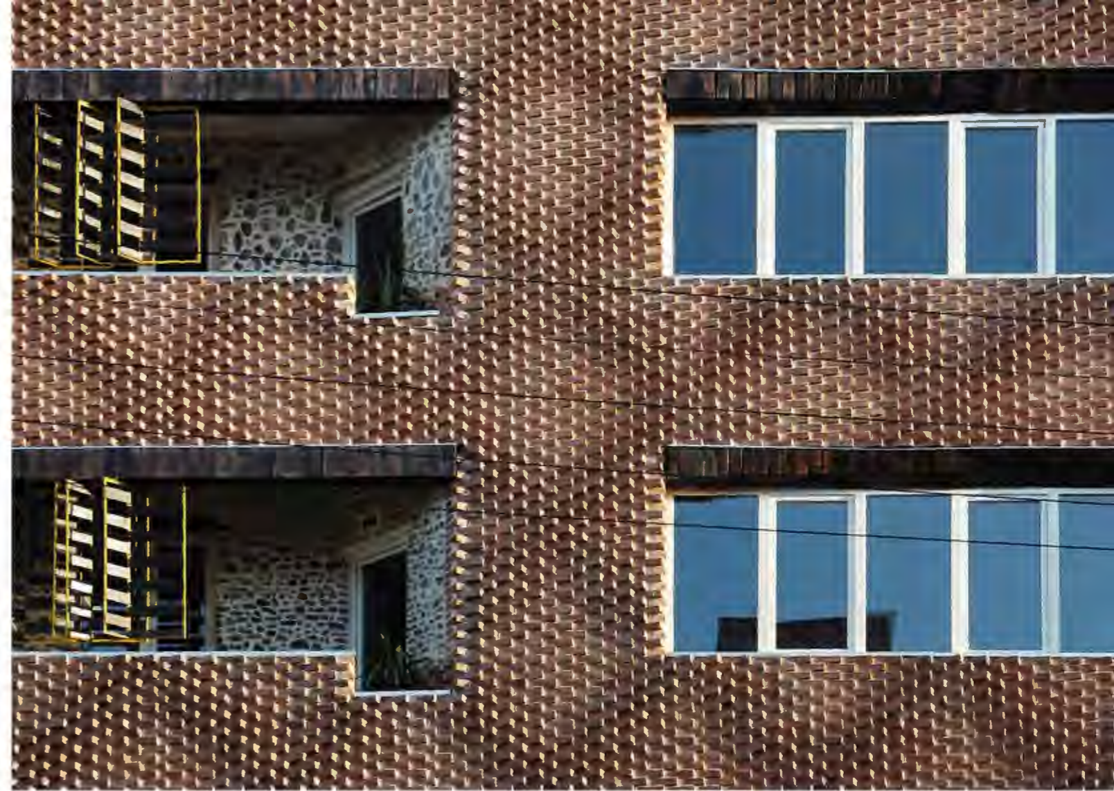
figure 94. Facade of APT NO.7
