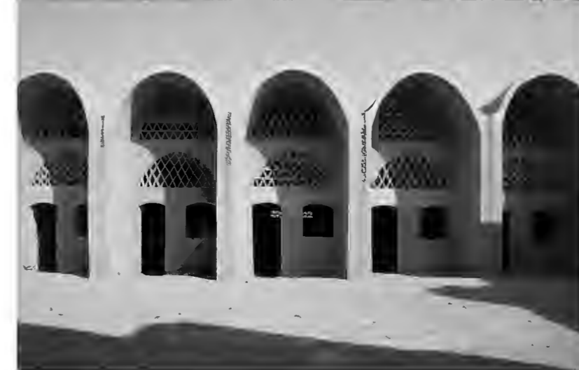
figure 86. He drew from traditional construction techniques, reused traditional forms of simple rural dwellings and used local materials such as mud. he builds modest and basic constructions for traditional Arab communities.
