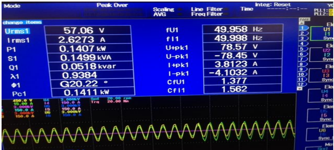
Figure 5.2 Reading from Yokogawa power meter.
