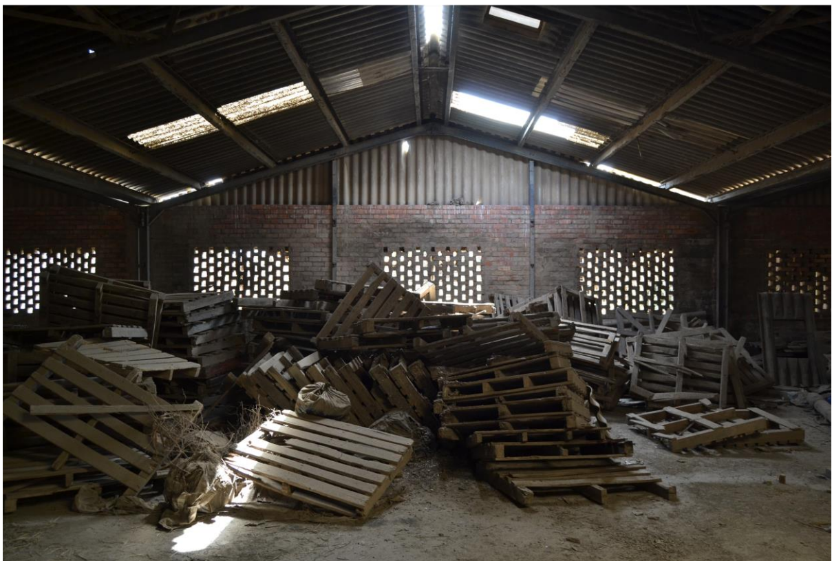
Figure 18: Interior images of buildings west wing with its collection of timber pallets (Author, 2023).
