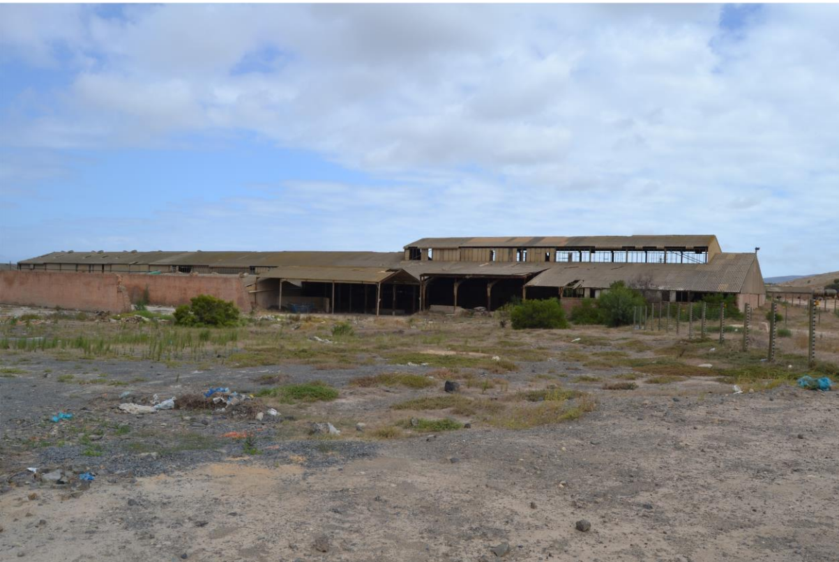
Figure 20: External views of the Northeastern section of the existing building (Author, 2023).
