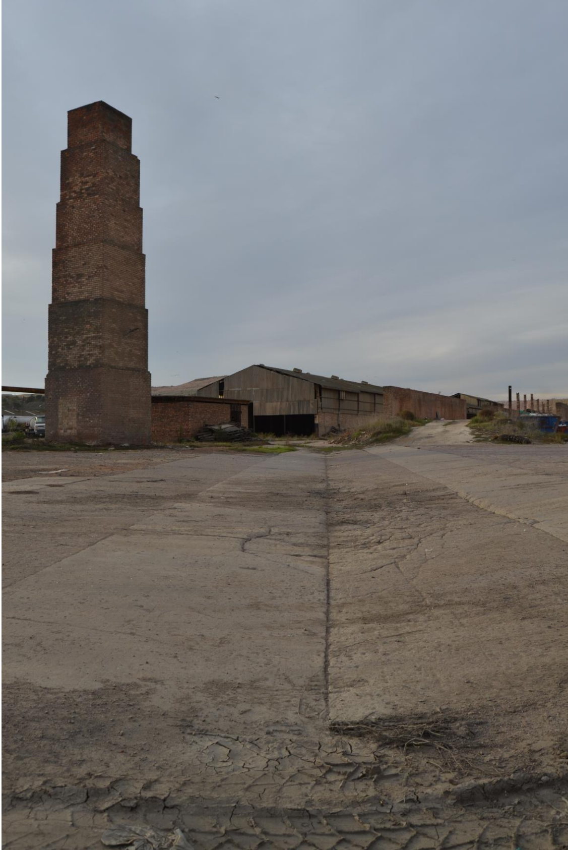
Figure 13: Existing, abandoned Clay Manufacturing Plant – Largest structure on site (Primary Building Focus) (Author, 2023).
