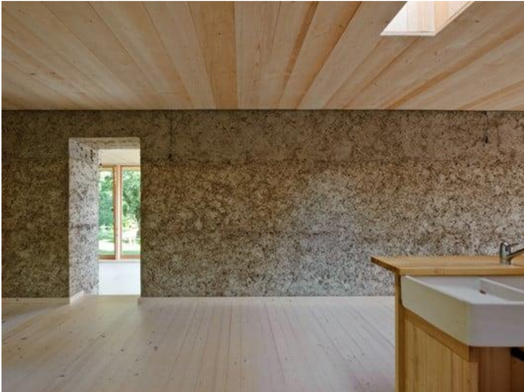
Figure 29: Wohnhaus Flury – View of one of the internal cob walls (Lewis et al., 2022).
