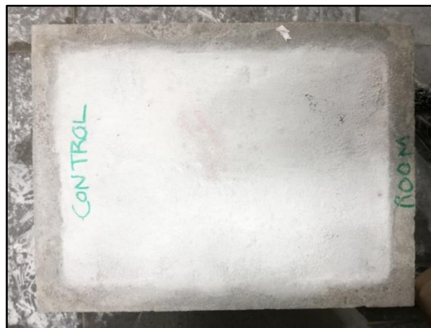
Figure 4-32: Control patch repair left under room conditions
