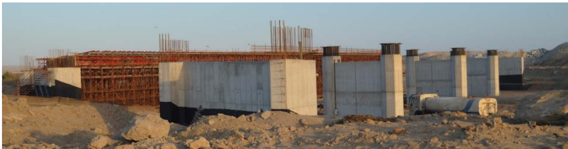
(b) Swakop river bridge piers and abutment
