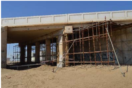
(a) Falsework erected under bridge
