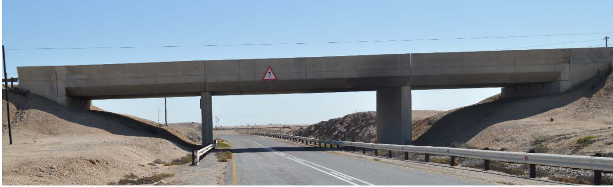
(a) B2 Bridge over Rosing Road and Rail
