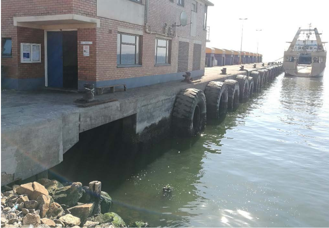
Fig. 6-2: Part of the small craft jetty structure
