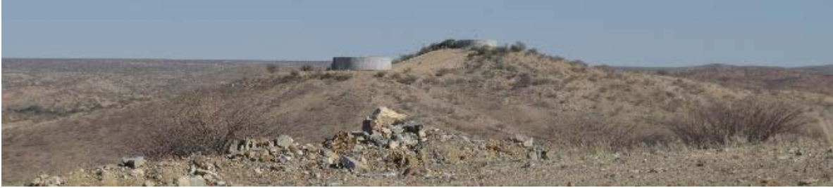
(a) Main supply tanks on the hill overlooking Usakos Town
