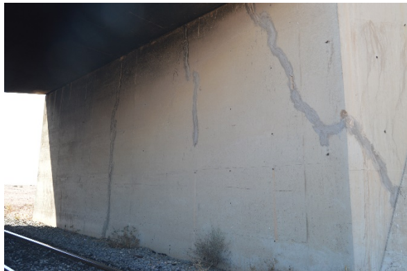
(b) Abutment wall with repaired cracks
