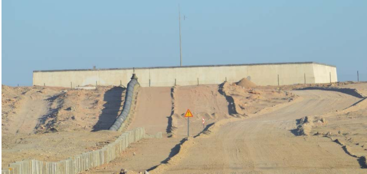
(a) Off C14 Water tank
