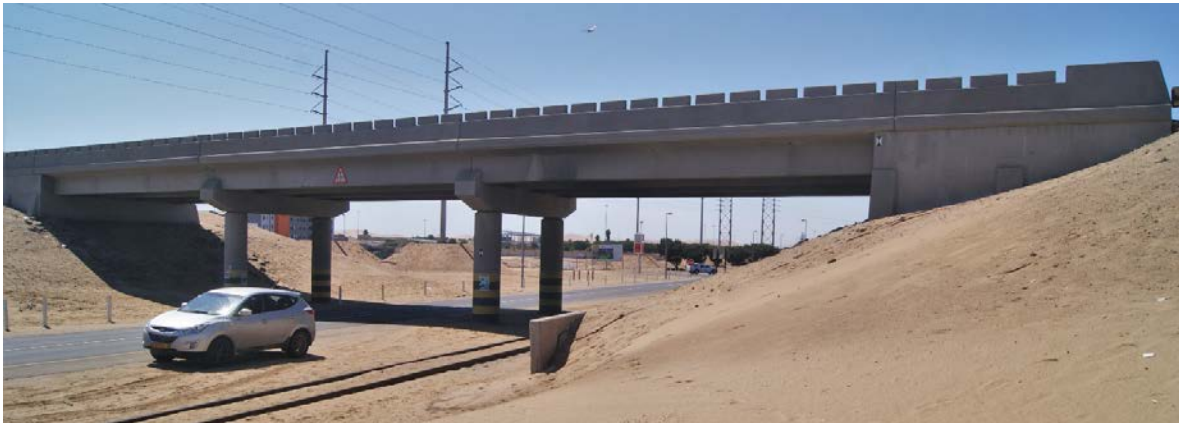
Fig. 6-8: Walvis Bay B2 Overpass Bridge
