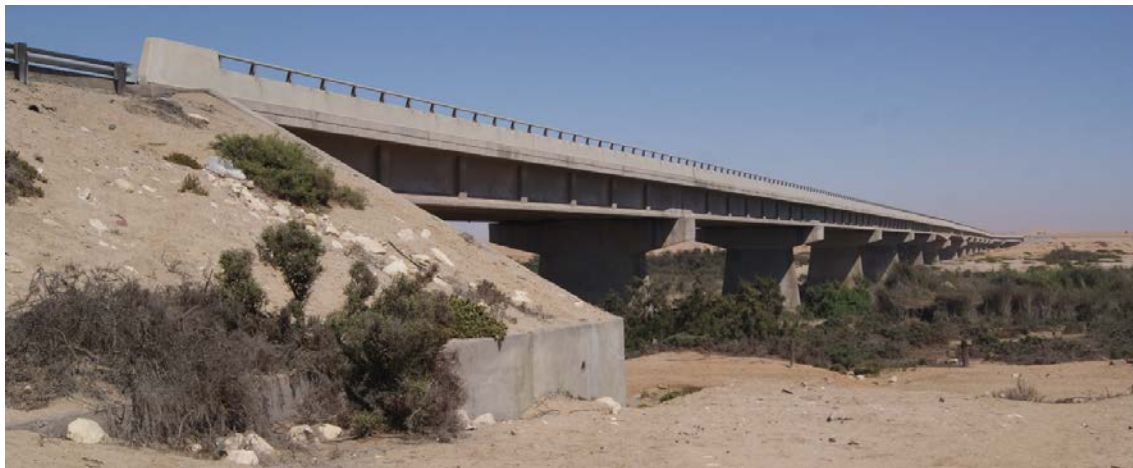
Fig. 6-10: Swakop River Bridge
