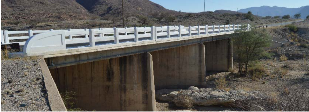
(a) Usakos East B2 bridge
