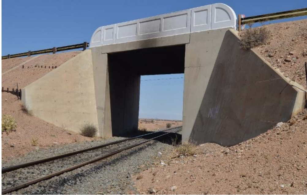
(a) Arandis Road over Rail bridge
