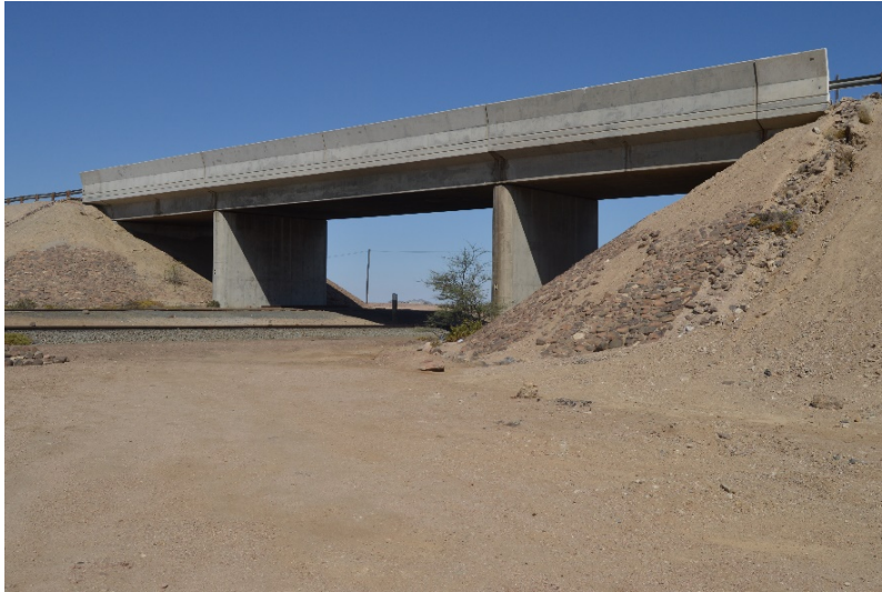
(a) Arandis Road Bridge over rail
