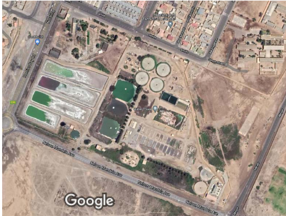
Fig. 6-16: Aerial view of Old Swakopmund Sewerage treatment works (Google map 2020)
