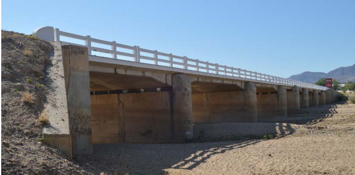
Fig. 6-23: Usakos west B2 bridge.
