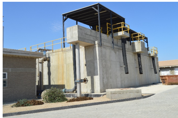
(f) Newly built lift station
