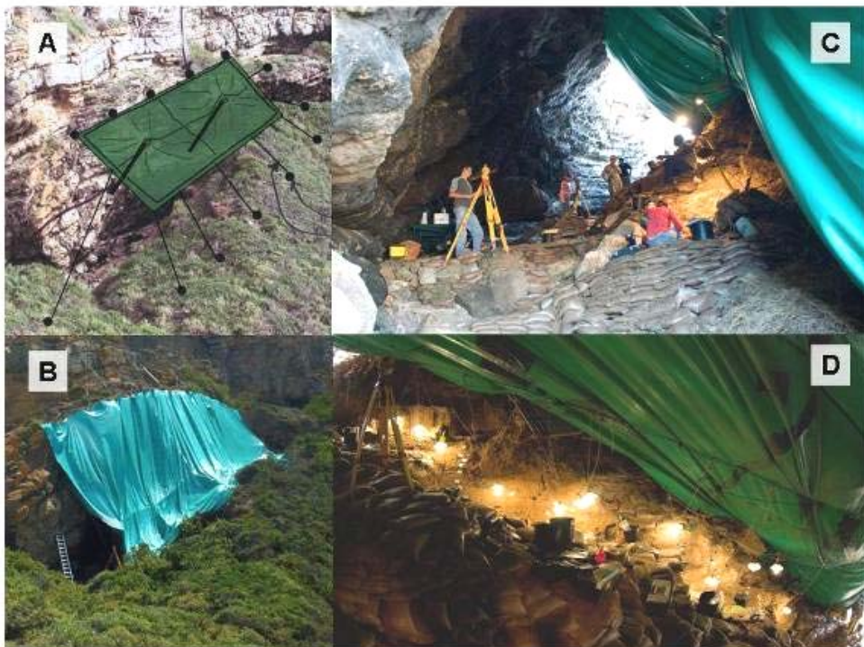
Figure 2. PP5-6 Sailcloth. A) as designed; B) installed 2007; C) PP5-6 view beneath sailcloth from south to north; D) PP5-6 upper Long Section view east
