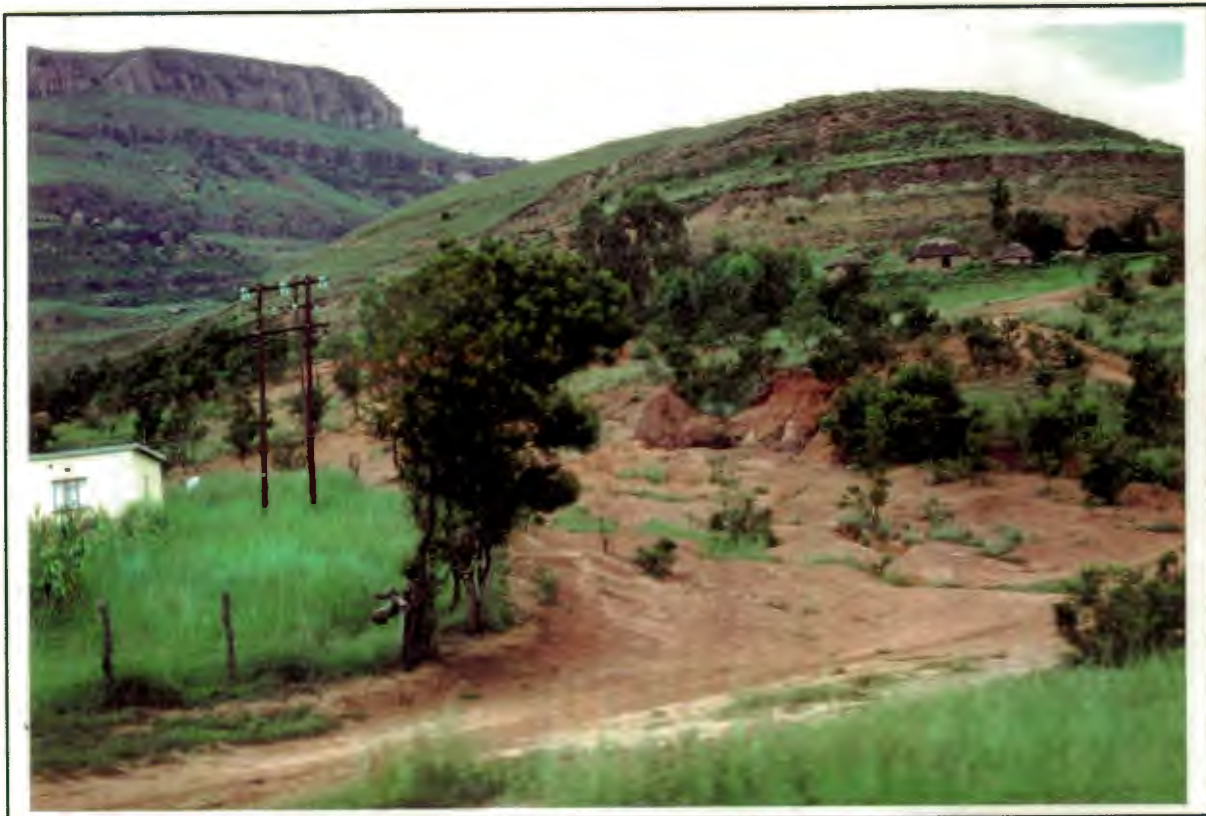
Plate 2.6: Severe gully and rill erosion along footpaths. Also note the alien tree infestation in the vicinity of the eroded areas.
