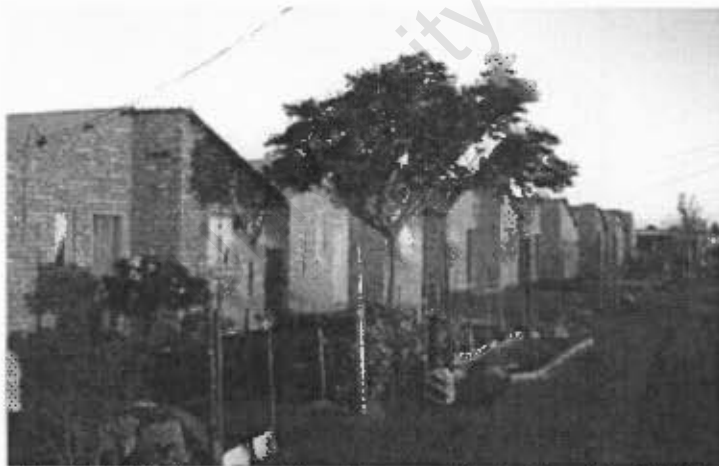
Figure 13: Kutlwanong Eco Houses, Kimberley, South Africa
