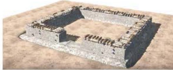
5) Bottles are arranged on foundation according to figure X configuration. Fishnet ropes are placed every half meter.
