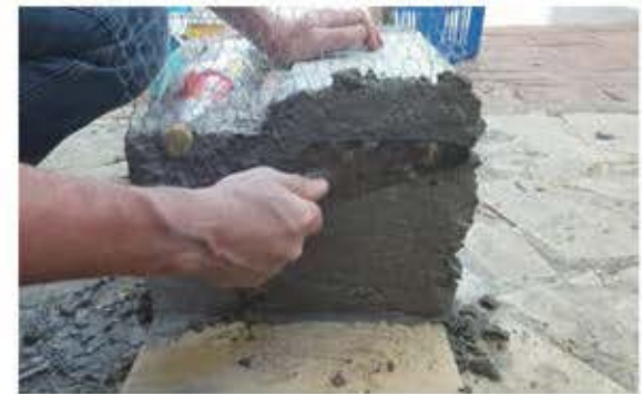
Build using above materials and chicken mesh reinforcement.
