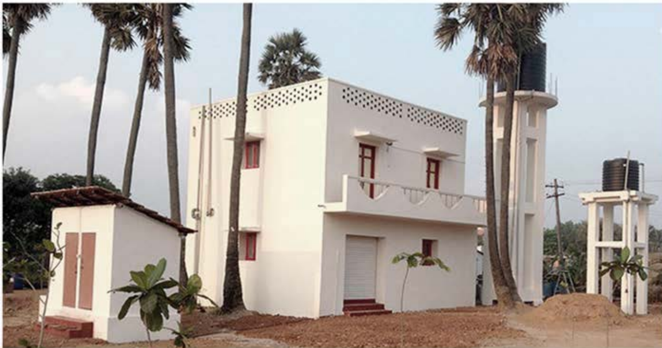
Figure X Redhills Forest Nursery, Chennai, India. The double story structure and 8m tall water towers are built with bottle bricks and uses fishnet & fishnet ropes for reinforcement. Source: https://samarpanfoundation.org/news/redhills-forest-nursery-relocates accessed 27/09/2017
