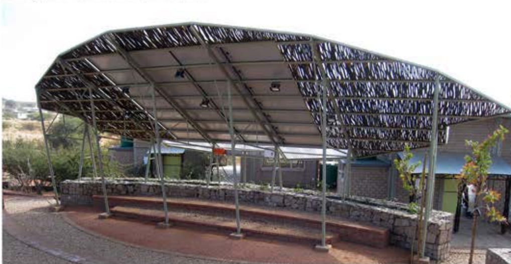
Figure X: Nina Maritz' Habitat Resource and Development Centre using reclaimed wood in between steel members as a shading device.
