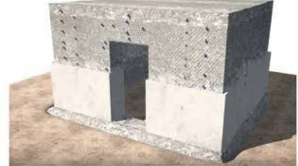
9) The walls are plastered and the fishnet is trimmed and melted with frame at the rod and window openings.
