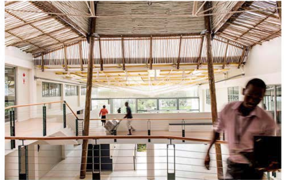
Figure X: Africa Centre by Eastcoastarchitects constructing a roof from reclaimed Eucalyptus poles, and thatching laths are used for shading and balustrades.
