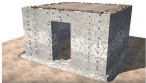
7) Once the height is achieved, fishnet is connected to the bottle caps on the outside surface, making the bottles one continuous surface.
