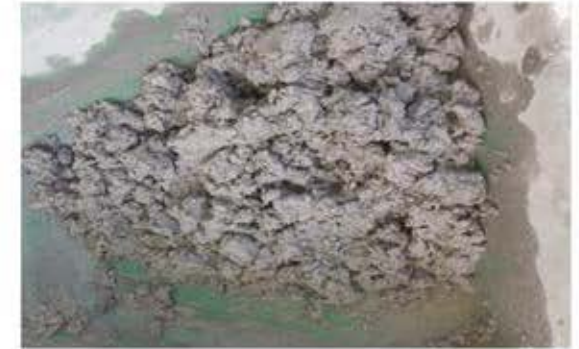
Prepare papercrete using paper pulp, concrete and sand.
