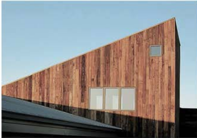
Top Figure X : BARNagain by In.Site-Architecture, using reclaimed timber as cladding. source: https://www.6sqft.com/ accessed 29/09/2017
