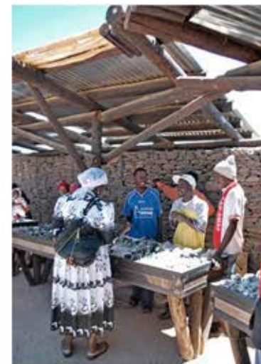
Figure X: Uiba-Oas Crystal Market by Nina Maritz architects using reclaimed invader trees as roof structure and support.
