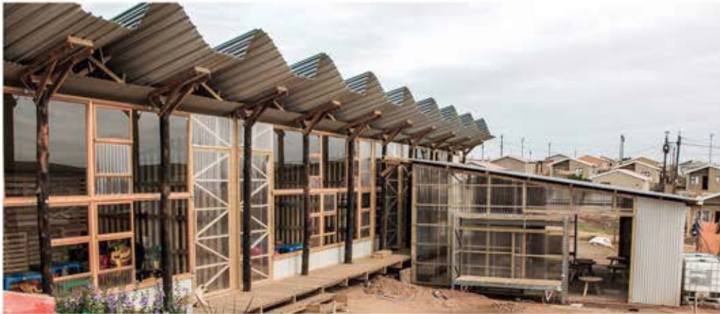
Figure X: Collectif Saga Architects' Silindokuhle Preschool in Port Elizabeth using eucalyptus trees and reclaimed wood as roof support.
