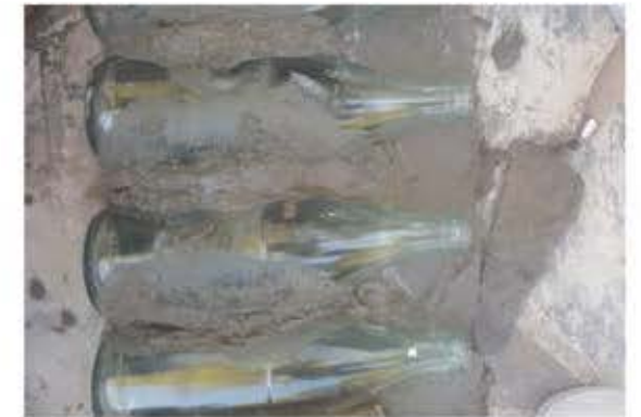
Prepare concrete mix and build using prepared bottles (brick substitute).
