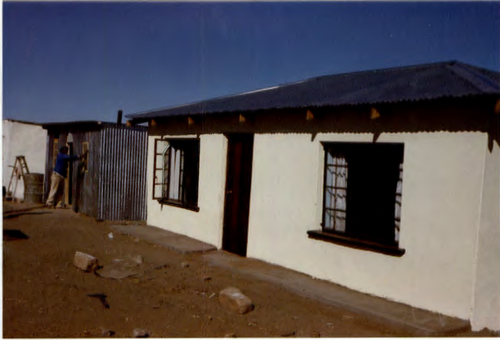
PHOTO 3: A new concrete brick and corrugated iron roofed house.
