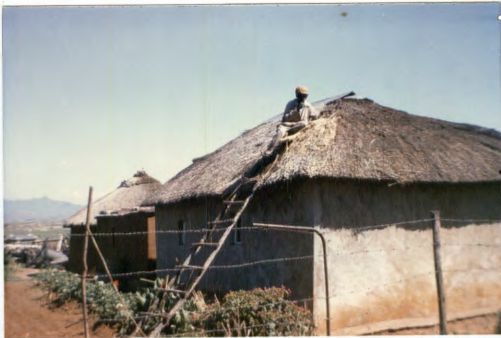
PHOTO 4: Mending the roof of a mud and thatch house.
