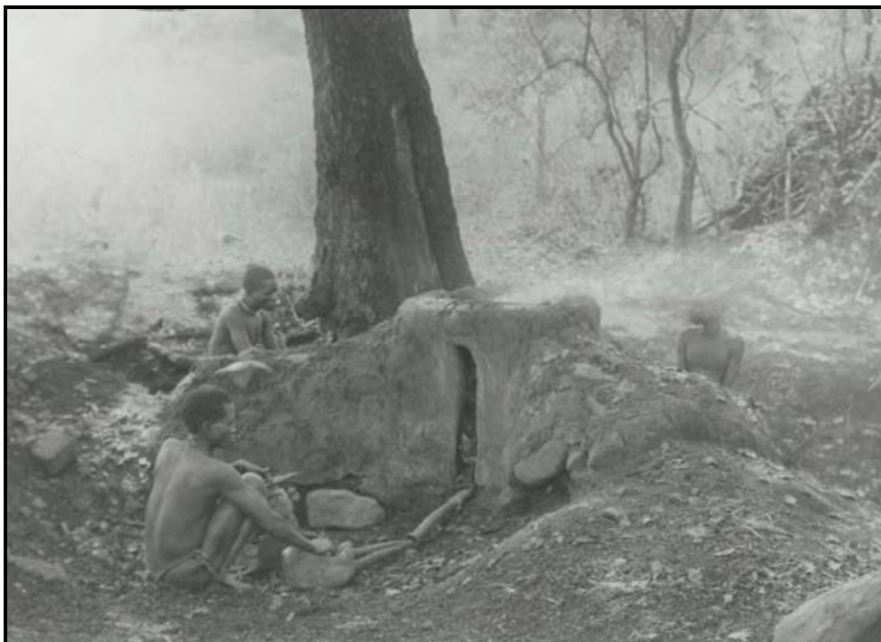
Figure 6: View of the iron production furnace photographed by H Gross in 1888 on the farm Schynshoogte, Soutpansberg (Macmillan, 1927).
