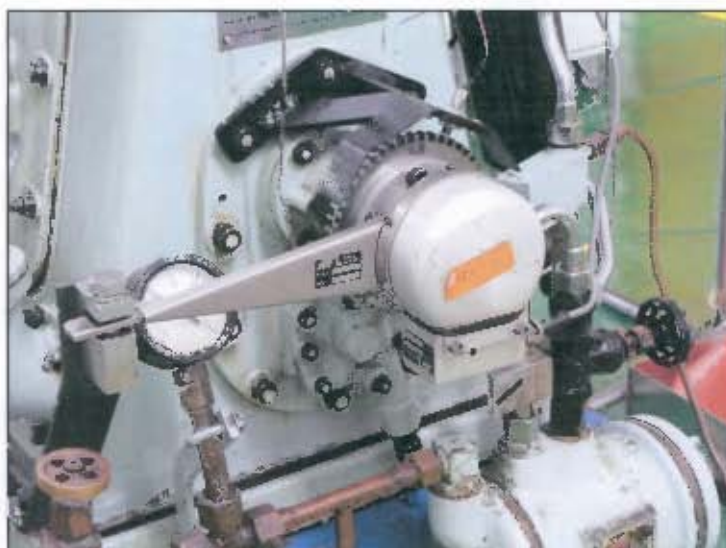
Figure 4-3 The crank angle encoder fitted to the engine.
