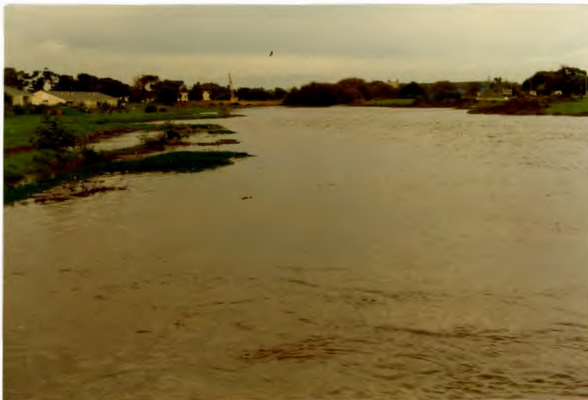
PLATE 21: Hartleyvale weir under flood.
