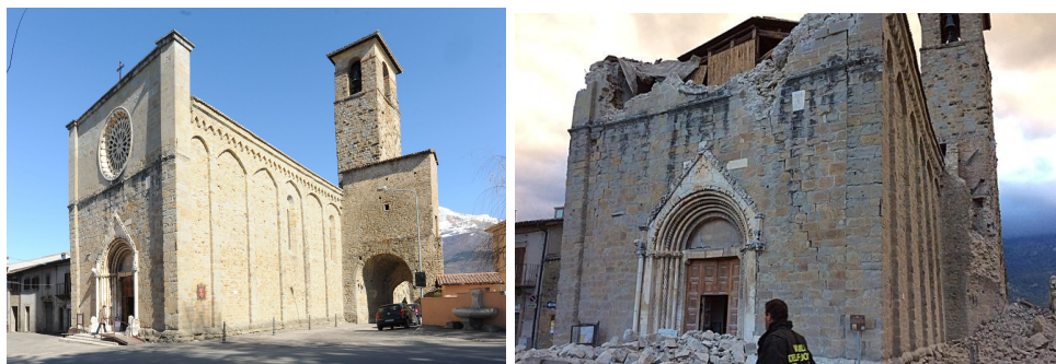
FIGURE 1.1: The Church of Sant’Agostino before and after damage
