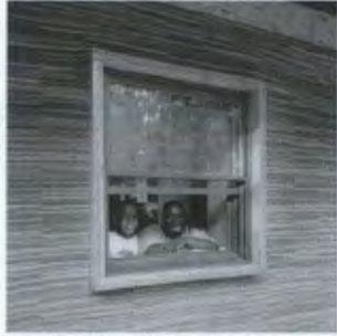
Figure 18: Lucy House, Rural studio. Source: www.ruralstudio.com Unused carpet tiles are dry stacked to make up load bearing walls. The tiles were held in compression by a ring beam to overcome horizontal instability.
