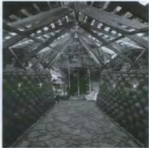
Figure 19: Yancey Chapel, Rural studio. Source: www.ruralstudio.com 900 tyres were stacked and filled with compacted earth to form walls. Vertical rebar bound the walls and provided horizontal stability.
