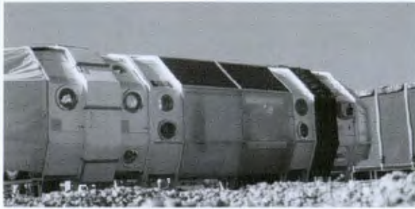
Figure 15: Miele Space Station, 2012 Architects Source: www.2012architecten.nl The reuse of discarded washing machines creates a new spatial type which is then appropriated in a variety of new ways, ranging from coffee bar, office and exhibition space.
