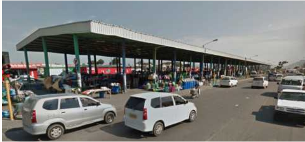
Street View of Nyanga Taxi Interchange (Google Earth) earth.google.com/web/.
