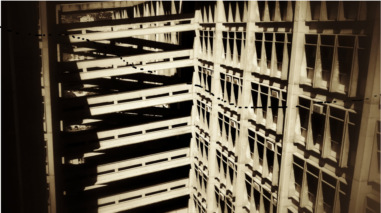
Concrete Walkways in the UERJ Education Building
