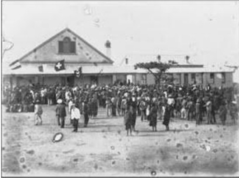
Figure 2: Picture of Elim Hospital in 1938 5
