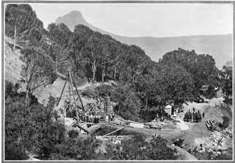
Fig. 07 Construction of the battery Site (Concrete working platforms)
