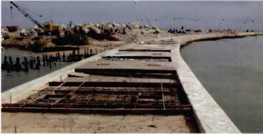
Figure 5-7: Reinstating of new slabs on Western Breakwater (Note existing capping beams)
