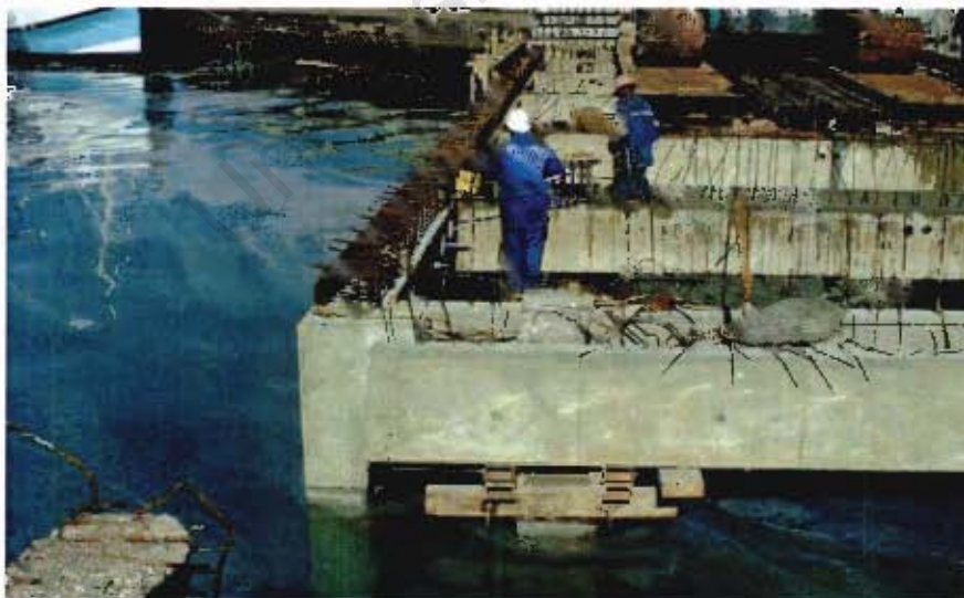
Figure 5-27: New works at Jetty 1, showing Precast Beam shuttering
