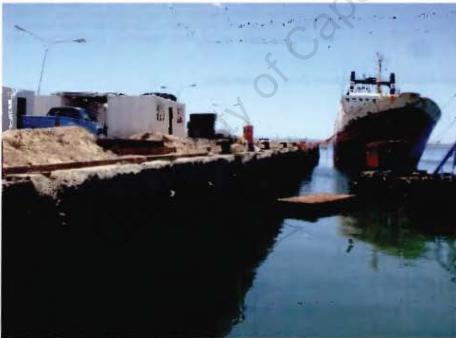
Figure 5-18: Edge beam of Government Jetty
