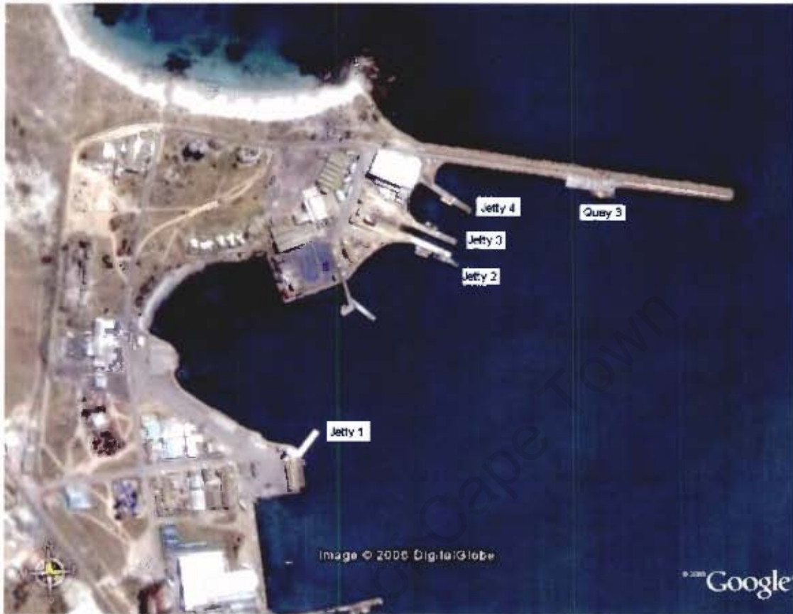
Figure 5-25: Aerial View of St Helena Bay Harbour (Google Earth, 2006)
