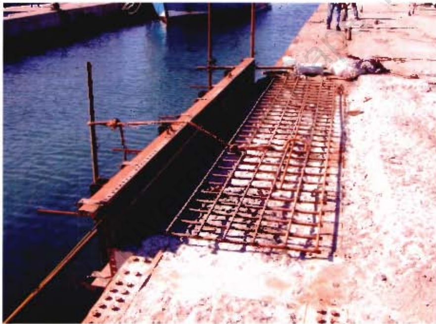
Figure 5-32: New reinforcement to Jetty 2 at St Helena bay
