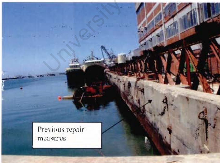
Figure 5-22: Trawler Quay showing 'strongback' girder
