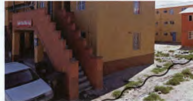
Figure 41: Soil erosion due to inadequate ground surface cover
