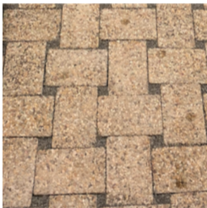
Figure 3-18: Pattern used for the exposed aggregate pavers (Cells I & J)
