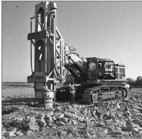
Figure 3.17: RIC machine operating (Van der Westhuizen and Parrock, 2010)
