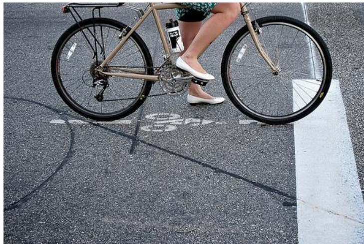
Figure 18: Inductive loop detector for bicycle detection (FDoT, 2019)
