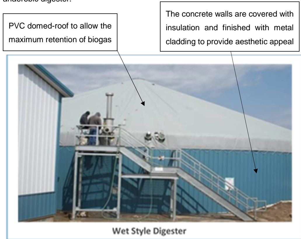
Figure 1: Photograph of a Typical Anaerobic Digester
