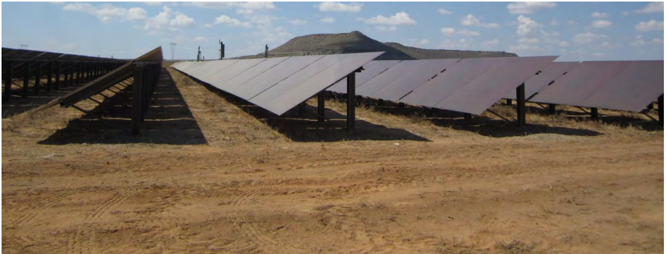
Figure 2.4 75MW PV Solar Plant under construction in Northern Cape (South Africa)
