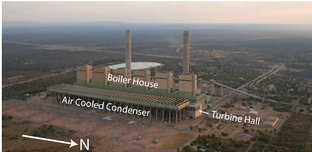
Figure 1.1: Matimba Power Station seen from the East with the A-Frame ACC units in the foreground
