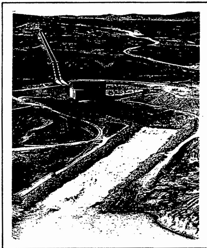
Figure 2.34 : Tekapo B power station discharging 100 \text{ m}^3/\text{s}
