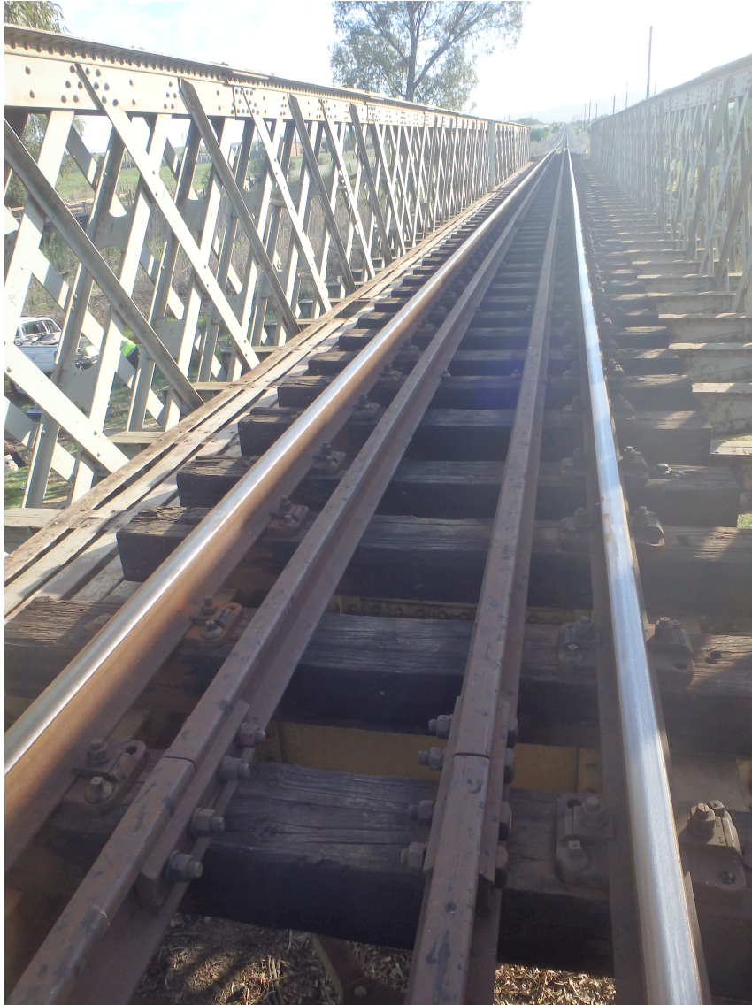
Figure 1.1: Open decked bridge
