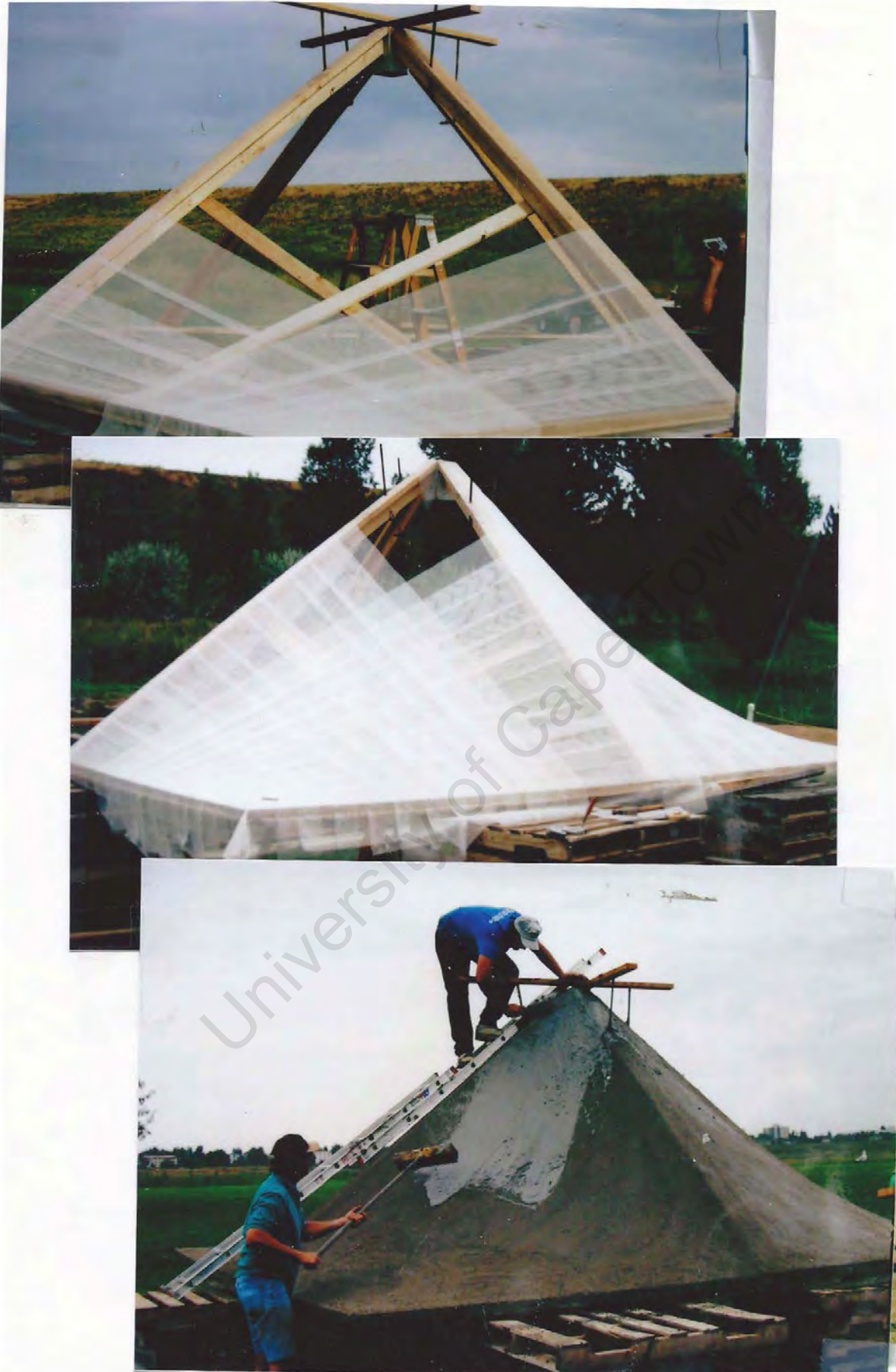
Figure 10: Image showing the construction of a hyper thin concrete roof (Osbbc.ca, 2013)
