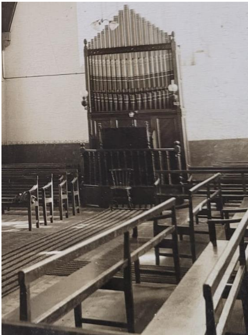
Figure 50: The German-made pump organ with its 19 pipes. (Source: Dutch Reformed Mission Church Wellington)
