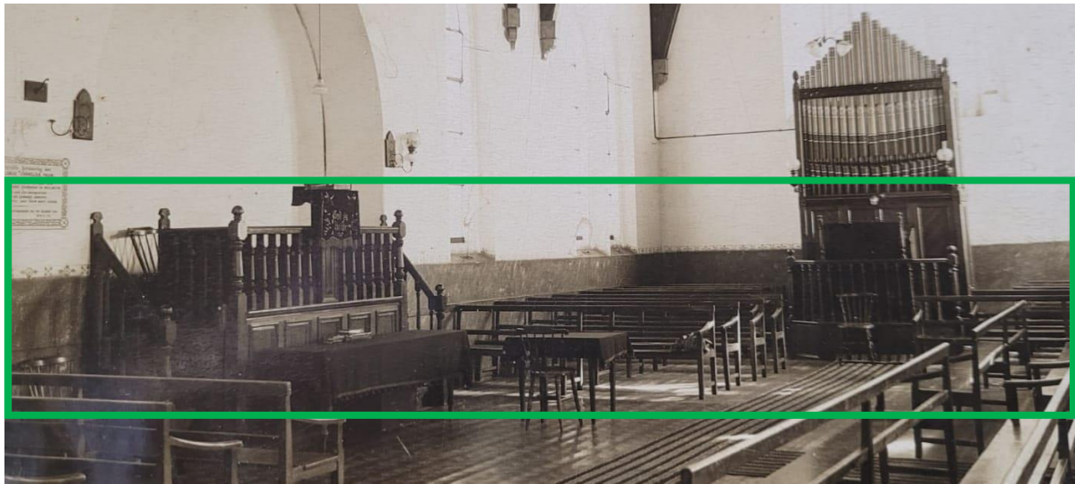
Figure 34: The green rectangular shape indicates the wooden varnished dado-panels which clad the inside walls. (Source: Dutch Reformed Mission Church Wellington)
