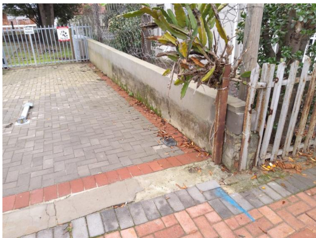
Figure 12: Original fence wall with remnants of original metal spike fence. (Photo: Pierre-Jeanne Gerber, 2020)
