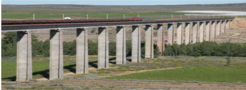
Figure 3.1: Olifants River Viaduct (Busatta & Moyo, 2018)
