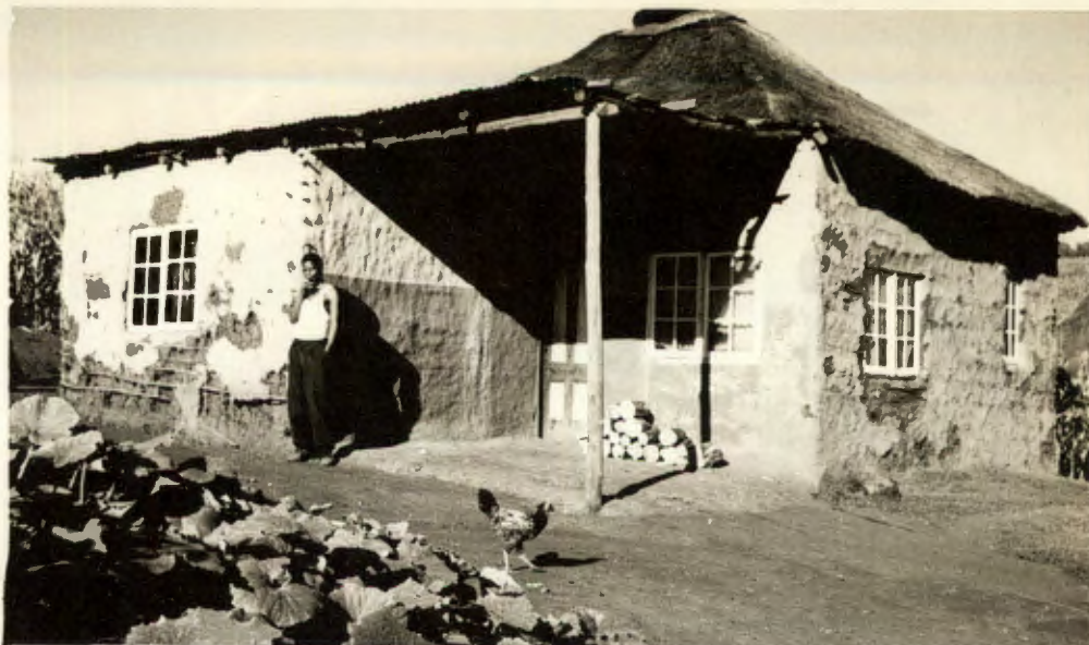
The home of Phineas Butelezi, Co. No. 6393/239, at Howick West. The house is constructed according to the type E1 plan. The house is in a fair state of repair.
