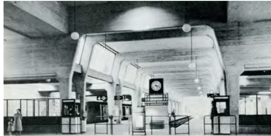
fig.94 - Concrete was shaping a new structural typology for train sheds in the time of modernism. Middlesex Station, Uxbridge. 1938. (source: Meeks C. 1957. Image by: London Transport Executive)
