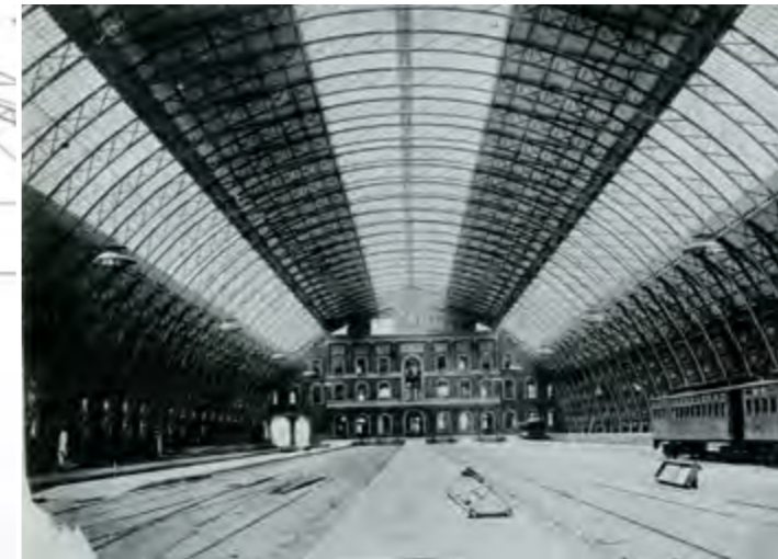
fig.90 - Arch without ties at New York's first Grand Central Station 1971. (source: Meeks C. 1957. Image by: New York Central System)
