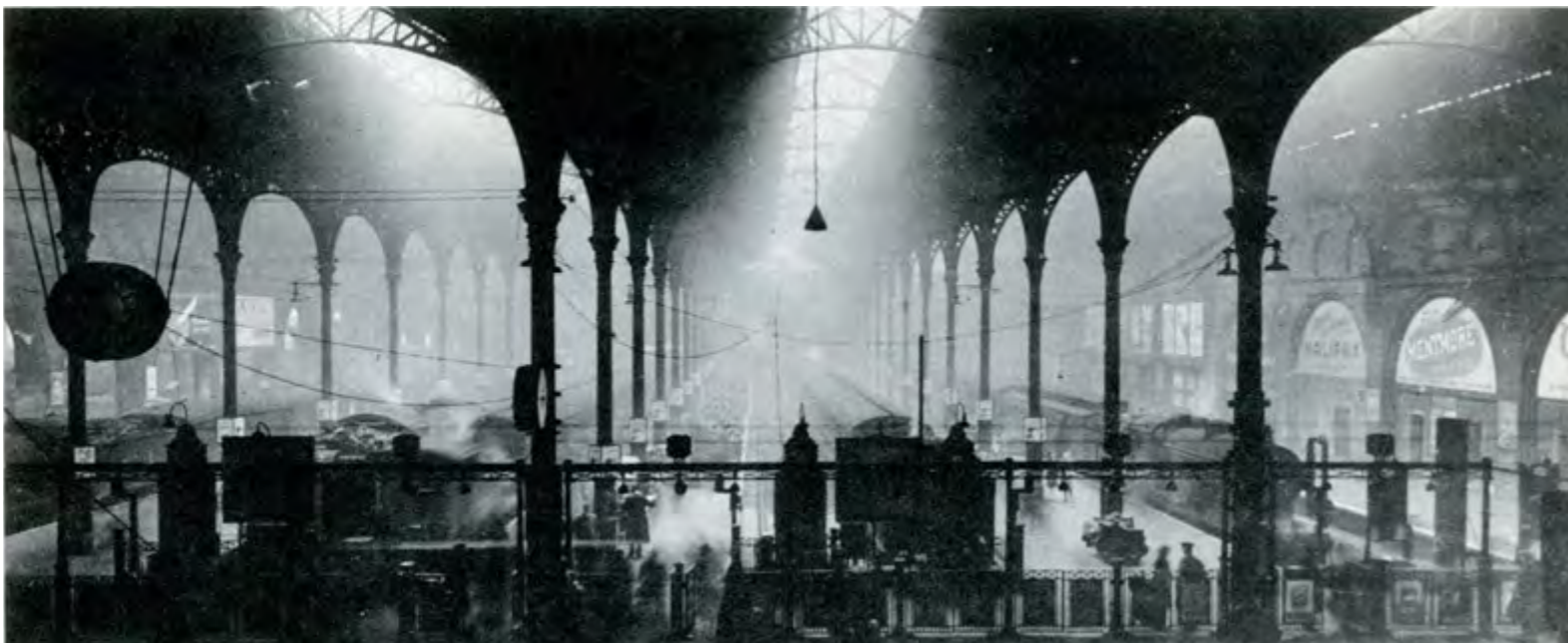
fig.92 - Image of the interior of a train shed showing the air quality and the need for natural light and ventilation. Liverpool Street Station, London. 1875. (source: Meeks, C. 1957. Image by: British Railways)
