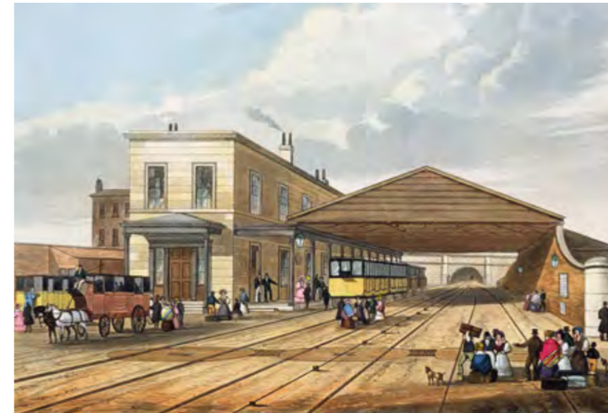
fig.85 - Crown Street Station, Liverpool, Britain, 1831, was the first station claimed to have a simple train shed. (source: Wikipedia. Image by: S.G. Hughes - T.T. Bury)
