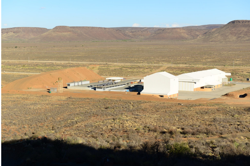
Figure 1.11: The Karoo Array Processor Building (KAPB) (to the left of the white integration buildings) at the Losberg Site Complex. [17]
