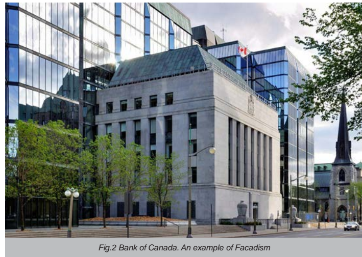
Fig.2 Bank of Canada. An example of Facadism
