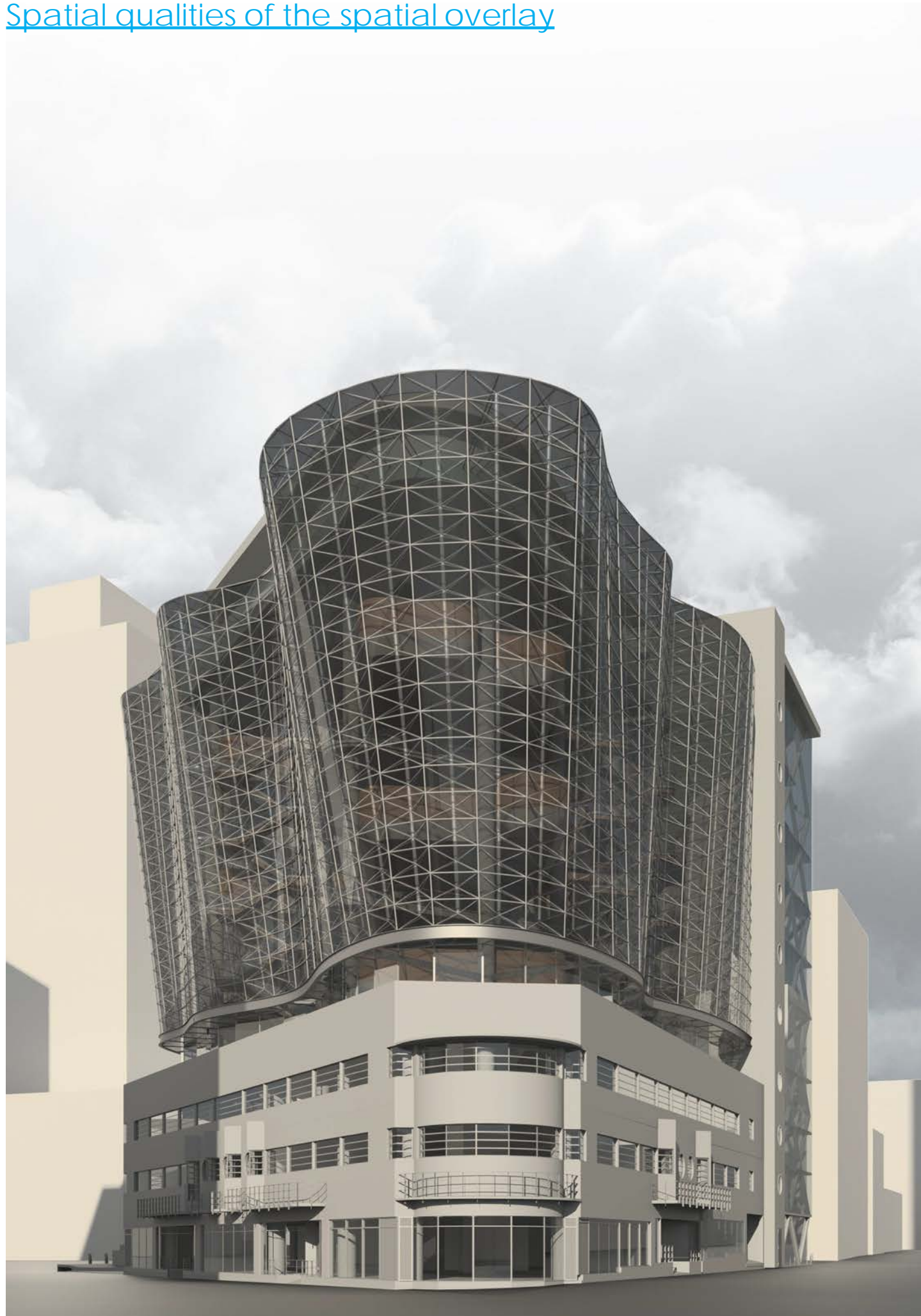
Fig. 50 Partially see-through glazing revealing the working pods and the columns
