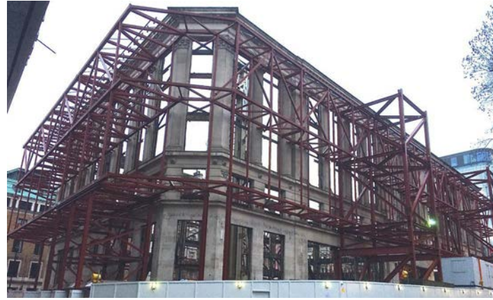
Fig. 1 Maintaining an existing facade while the interior is gutted
