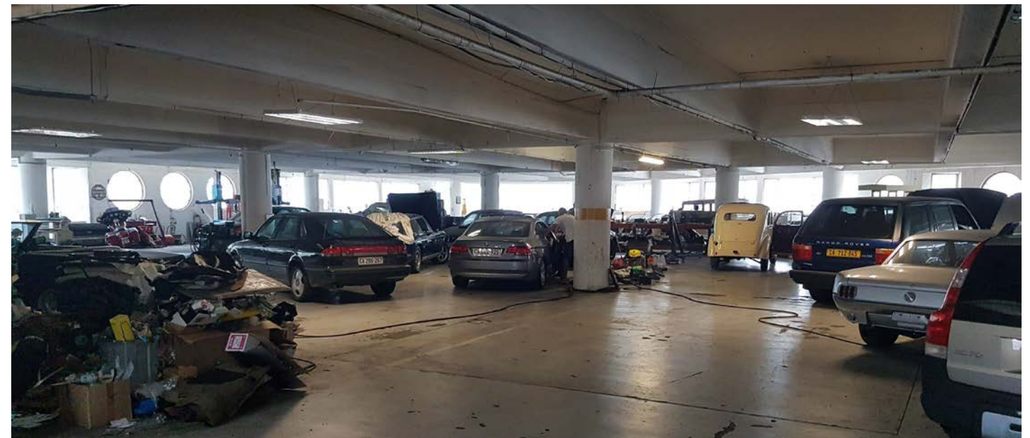
Fig. 13 Photograph of first floor above ground level (2017)
