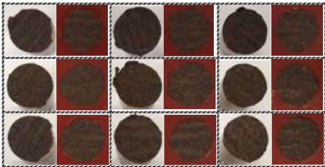
Figure 59: All NC1 samples test sites showed cohesive failure in the converted corrosion product underneath the coating, each row is a sample, and the dollies are on the left of the corresponding test sites.
