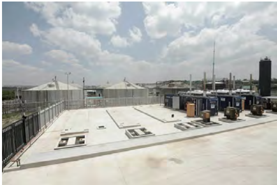
Figure 40. Johannesburg Water Northern Wastewater Treatment Works in Diepsloot.
