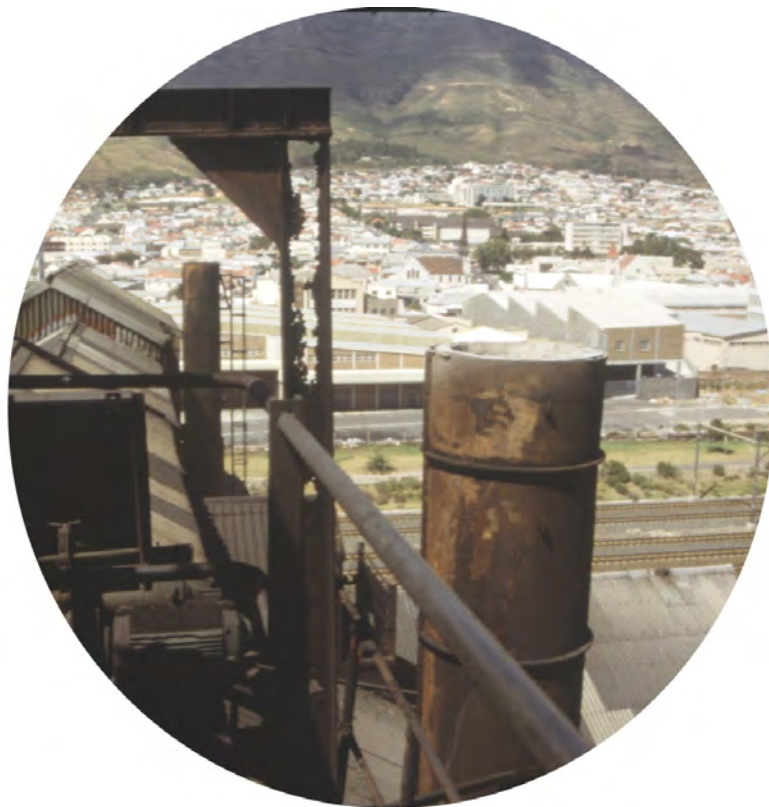
Figure 11. View of Woodstock and Devils Peak from the a gasworks structure Image from David Worth
