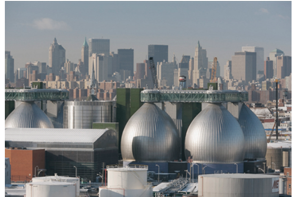
Figure 39. Newtown Creek Wastewater Treatment Plant, Brooklyn, New York
