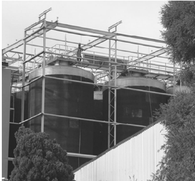
Figure 41. Biodigester at South African Breweries, Cape Town.
