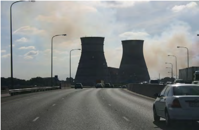
Figure 1. The now demolished cooling towers, Cape Town This is a missed landmark that many have grown a fondness for http://blog.africabespoke.com/cape-town-international-airport-upgrade/
