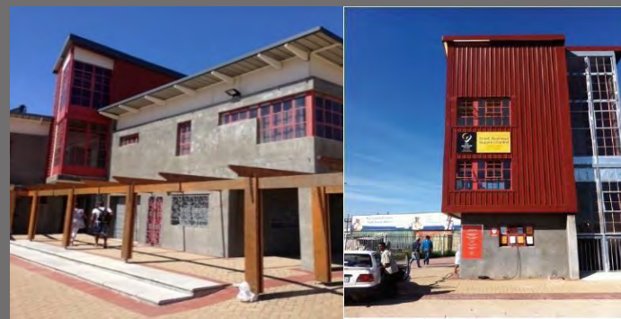
Active Safe Boxes and Low Cost Community facilities (Source: VPUU, 2012)
