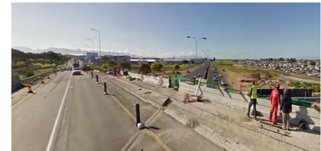
Figure 8.7 Airport Approach Road over N2 facing South East (Source: Google Street View, 2015)
