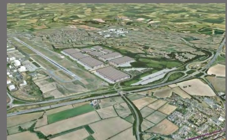
Grow Houses alongside airport runway (Source: Argent, 2015)
