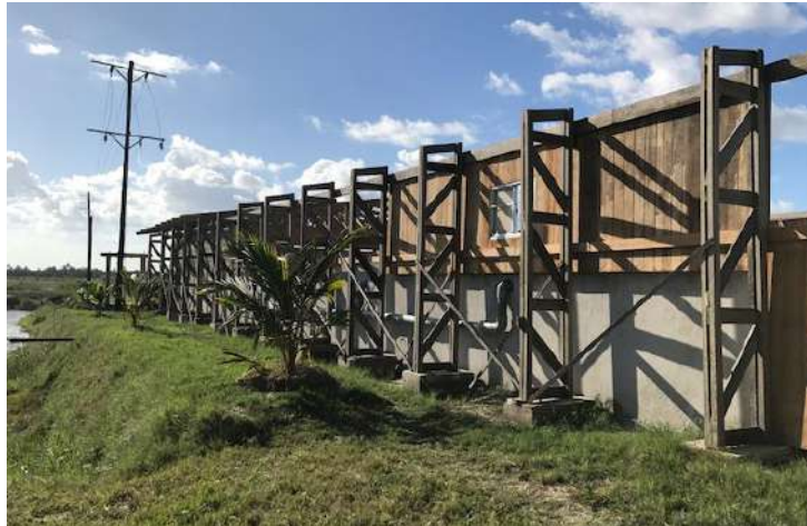
Figure 12: Coconut timber structure the author worked on. Its application is in the columns, the panels and the trusses. All the elements are prefabricated at the forest centre and assembled on site. Fish Farm, Beira.
