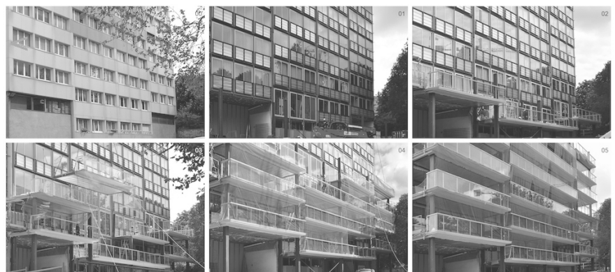
Figure 5: Prefabricated concrete and steel construction system, that was installed while residents lived in the building, Tower Bois le Prêtre
