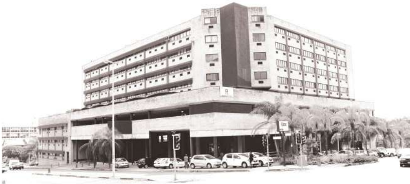
Figure 41: View from top of Bell Street (South view)
