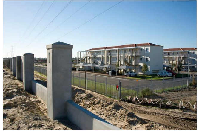
Figure 6.8: Apartments in case study 3
