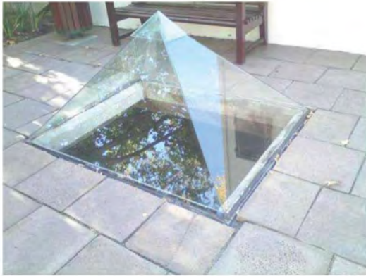
Figure 40 Glass skylight in the ground [author 2013]
