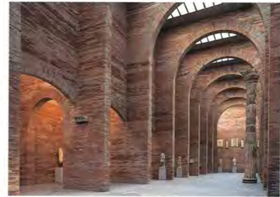
Fig 67 Museum of Roman Art elongated modular brick arches with concrete structure [Rafael Moneo, opposing forces PDF,2013]
