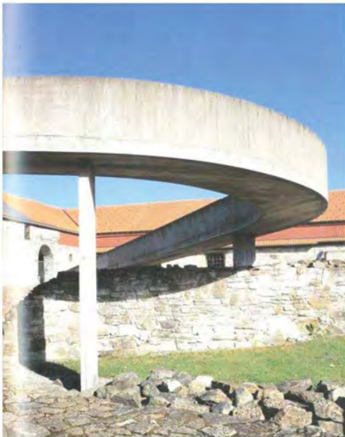
Figure 34 A concrete curved slope passes over the ruins and into the building [a+u, 1999:47]
