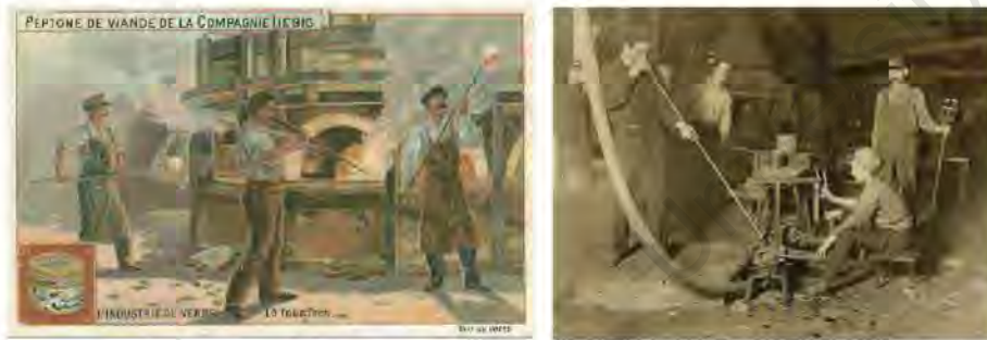
Fig 78 Glassmaking 1800's mouth blown process and 19th c. machine process [sha.org 2013]
