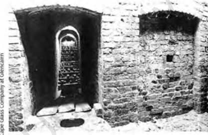
Fig. 14 A cross-section of the underground of the main tank showing a representative chamber of brick chamberwork (see fig. 15). A brick-lined chamber with a small taper iron pipe in on the right.
