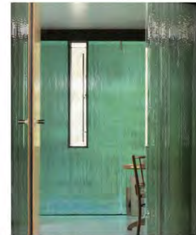
Fig 66 Laminata House exterior has vertical stacked glass sheet structural walls, Interior quality of light, vertically stacked glass sheet walls [Richards, 2006:194]
