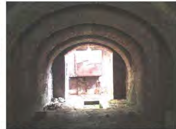
Fig 68 Main central Furnace Chamber brick arches supporting the tank at Glencairn [author, 2013]
