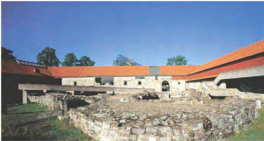
Figure 33 Courtyard with the Hamar Fortress ruins [a+u, 1999:46]
