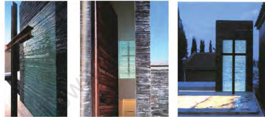
Fig 65 Stacked glass strips and slate, Mausoleum in Spain [Detail, 2004:362]
