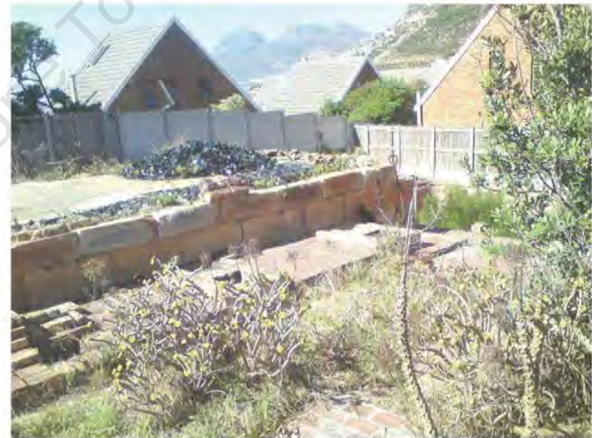
Figure 25 Neglected ruins of Cape Glass Company site [March 2013]
