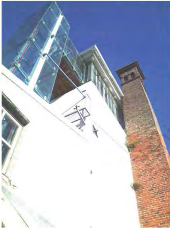
Figure 38 Brick chimney and glass elevator shaft [author 2013]
