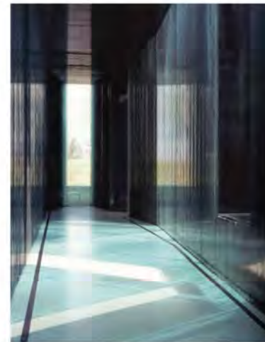
Fig 66 Laminata House exterior has vertical stacked glass sheet structural walls, Interior quality of light, vertically stacked glass sheet walls [Richards, 2006:194]
