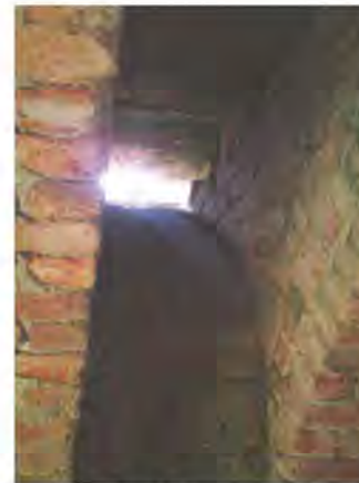
Fig 68 Main central Furnace Chamber brick arches supporting the tank at Glencairn [author, 2013]
