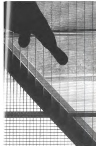
Figure 94 Steel grated platform [A Ferre, 2007:143]
