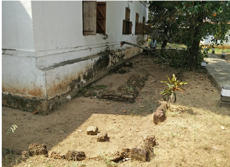
Photograph 13: Excavation showing original foundation of Paravur synagogue. Photograph by Mark Aranha, January 2018.
