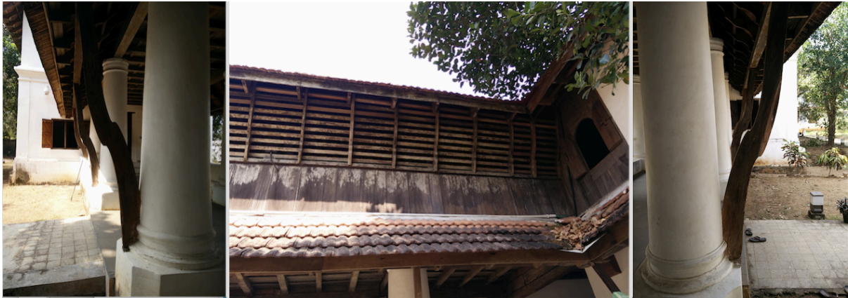
Photograph 17: The outside of the boat-room, flanked by pillars and wooden ship-ribs supporting it. Photographs by Mark Aranha, January 2018.
