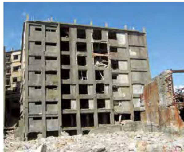
No. 30 and No. 31 Apartment Buildings
